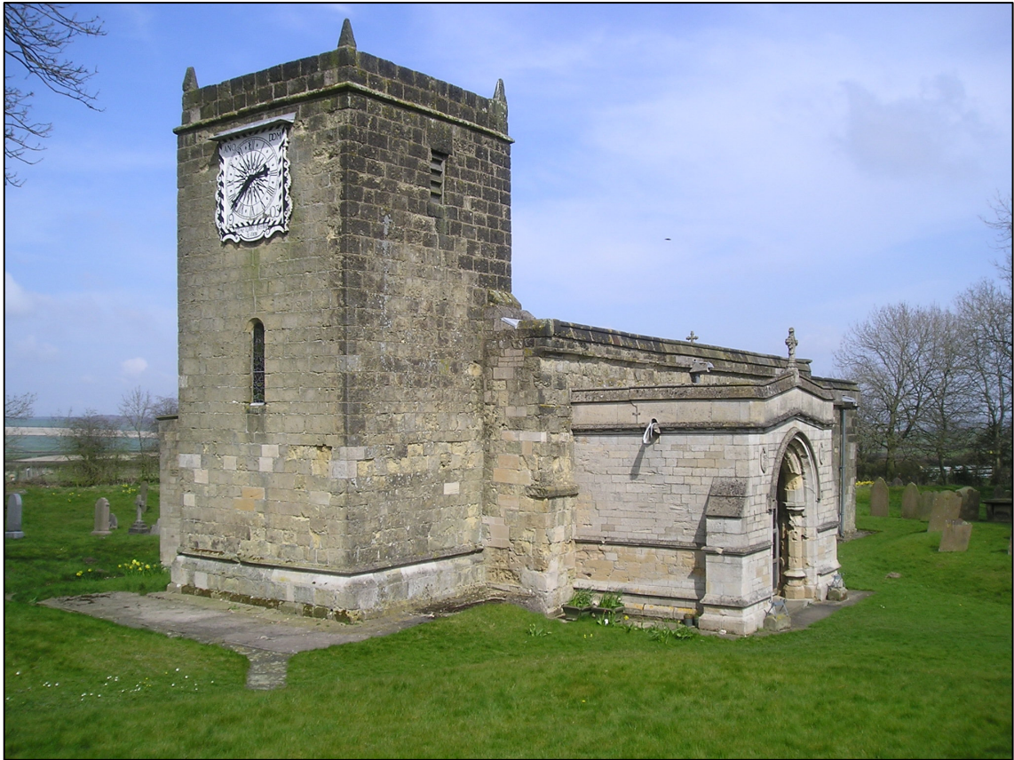
Plate 1: General view of St Mary's church, looking north-east.
