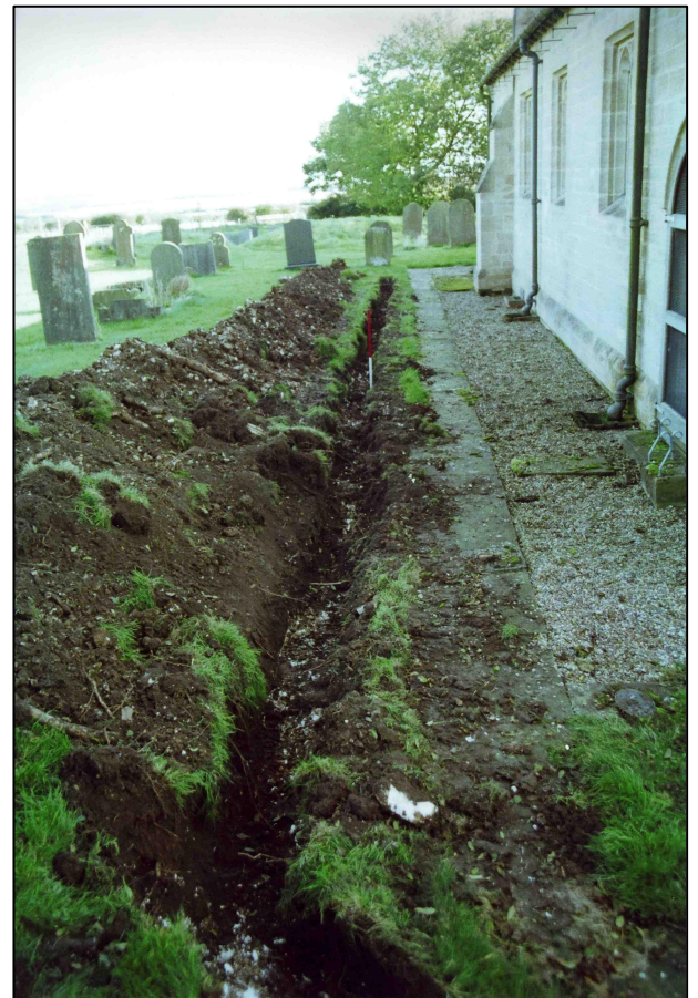
Plate 3: View of trench parallel to north aisle, looking east.
