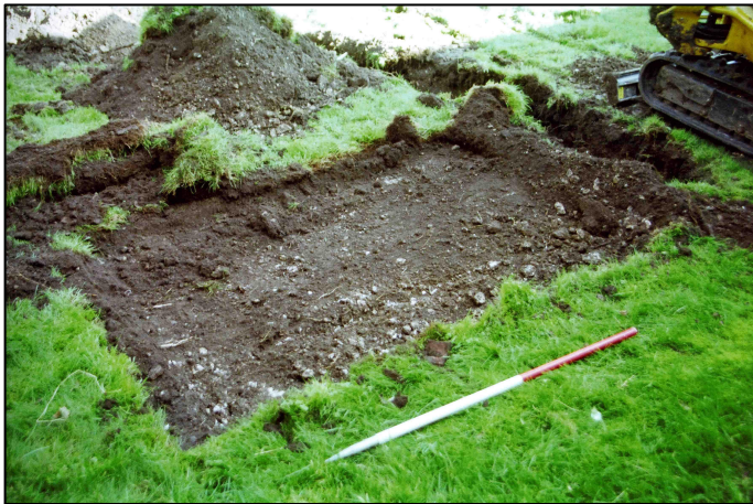
Plate 2: Excavated base for oil tank, looking NE.
