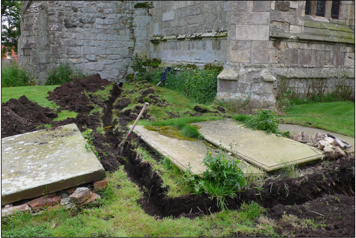
Plate 1: Northern section of drainage trench under excavation, looking east.
