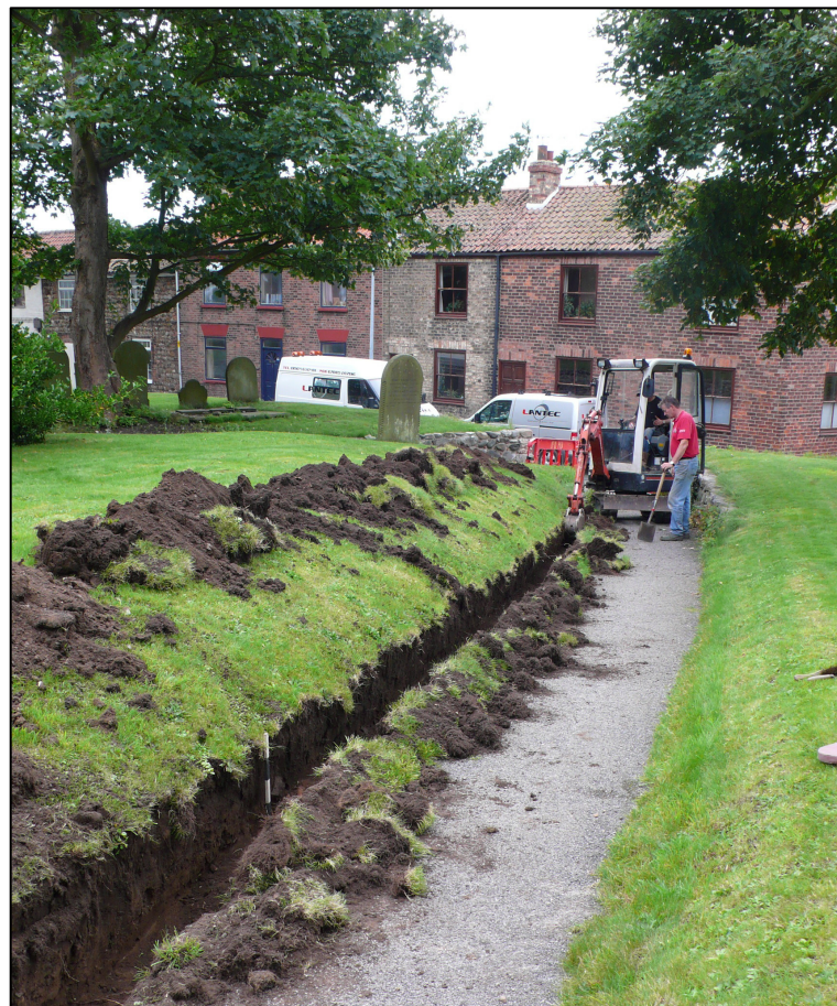
Plate 2: Southern section of drainage trench under excavation, looking south-east.
