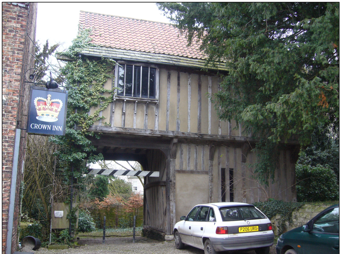
Plate 4: Bolton Percy Gatehouse, south elevation, looking north-west.
