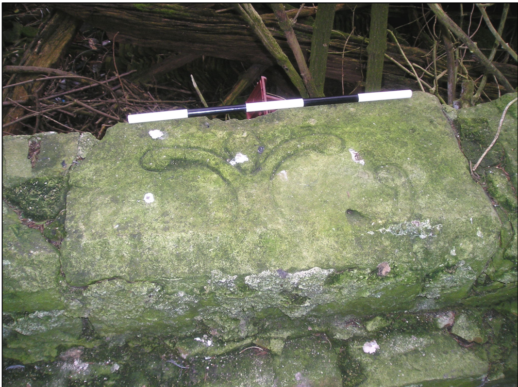
Plate 7: Reused coffin lid fragment on north plinth wall, west side of gatehouse.
