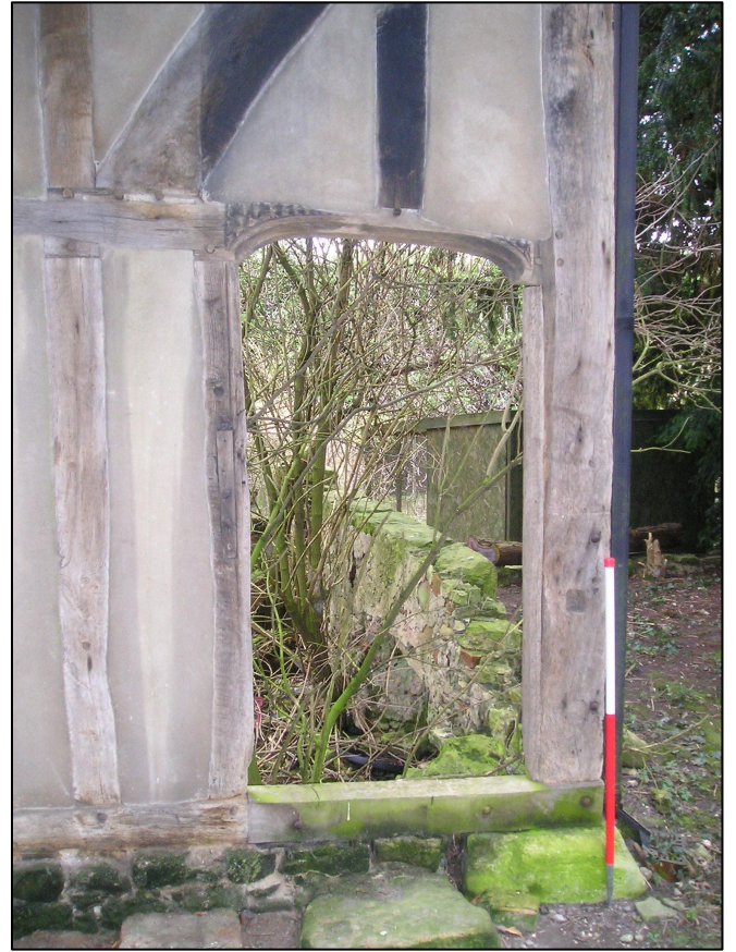
Plate 6: Doorway at north end of west side of passage, looking west.
