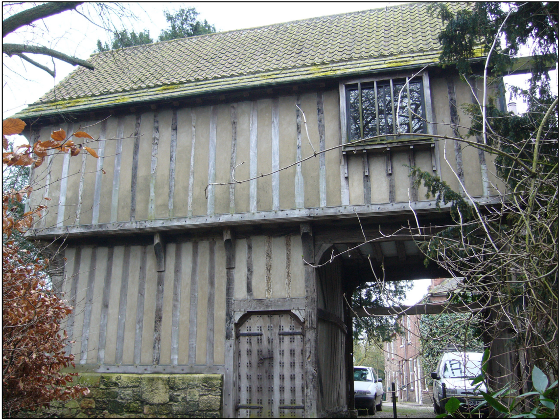
Plate 3: Bolton Percy Gatehouse, north elevation, looking south-east.
