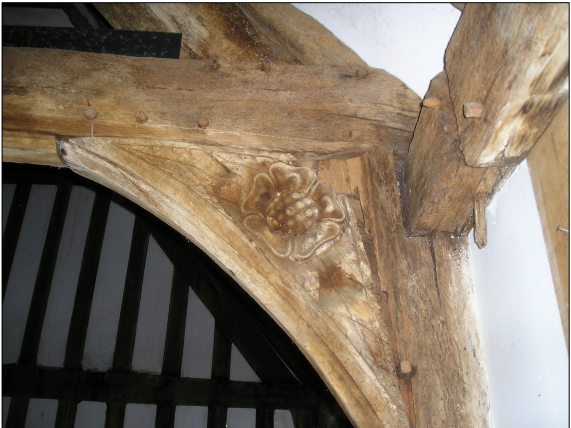
Plate 9: North knee-brace, east face of west truss, looking west.
