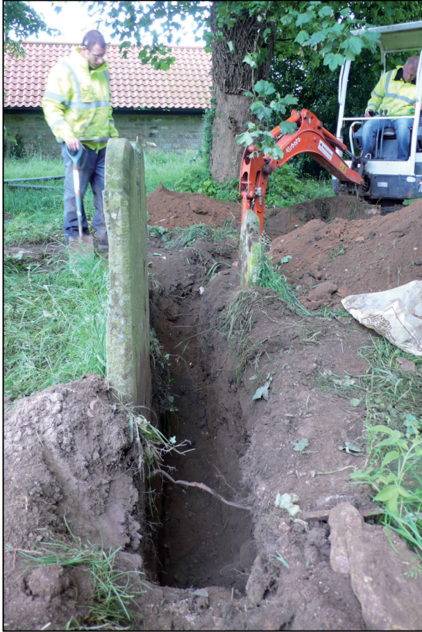
Plate 1: Trench excavation in progress, looking S.
