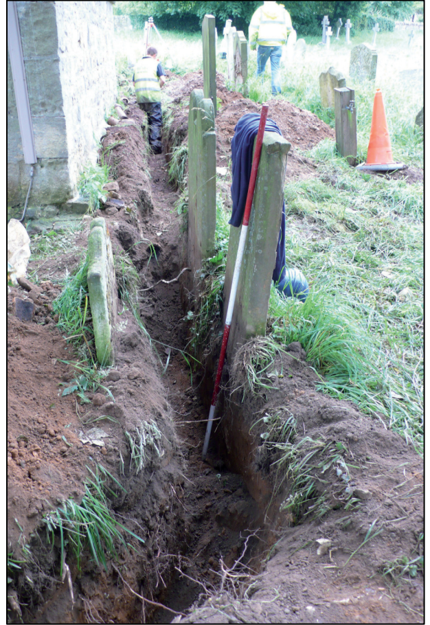
Plate 2: Excavated drainage trench, looking N.
