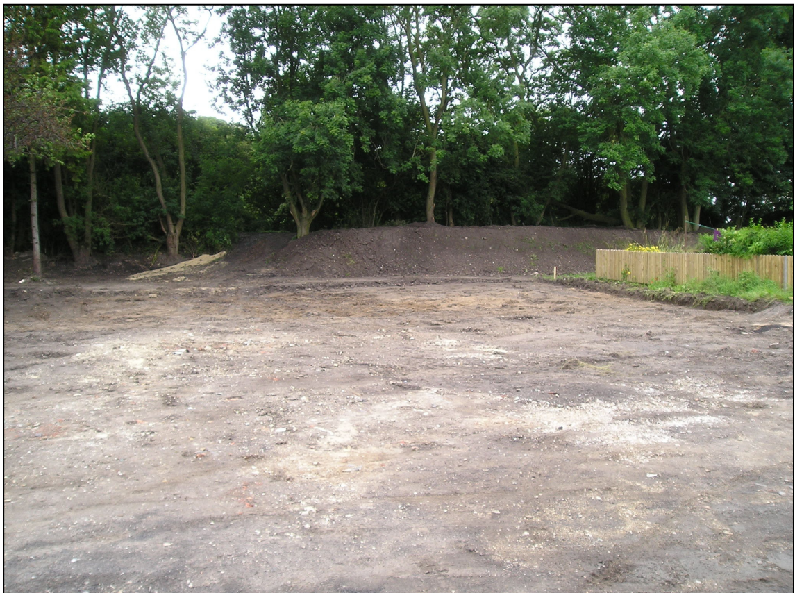
Plate 3: Car park area following topsoil stripping, looking south-east.
