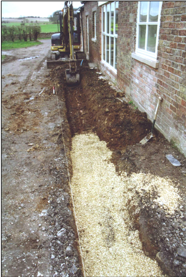
Plate 1: Trench 1 under excavation, looking north-west.
