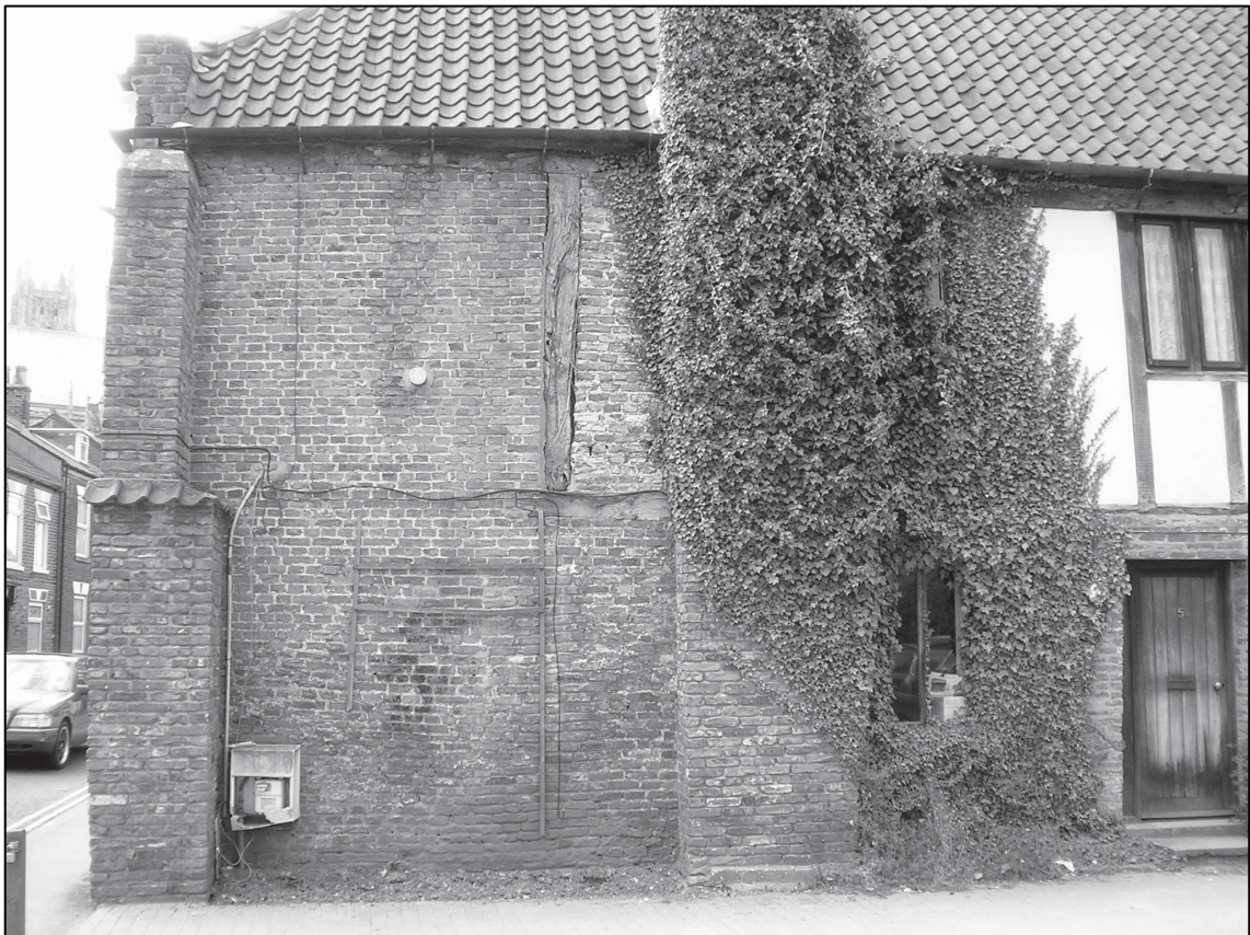
Plate 4: South end of east external elevation, looking north-east.
