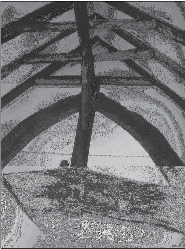
Plate 6: Northern surviving roof truss, looking north.
