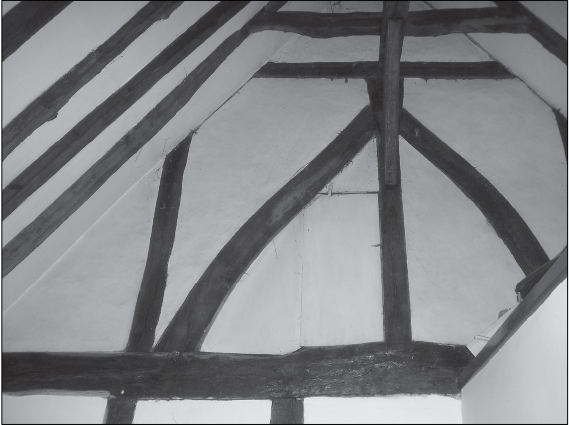
Plate 5: Frame of internal partition wall, looking north.
