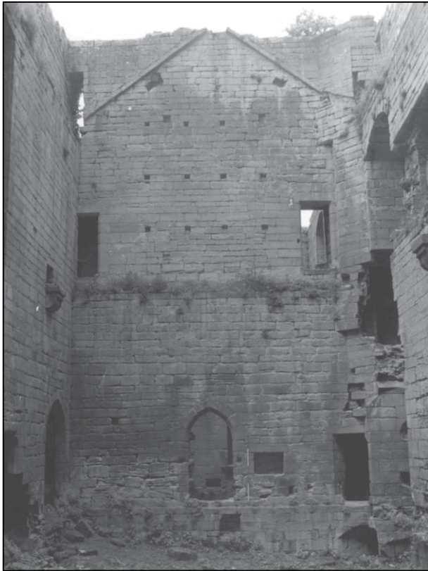
Plate 26: North internal elevation of hall block (elevation 19) (May 2000).
