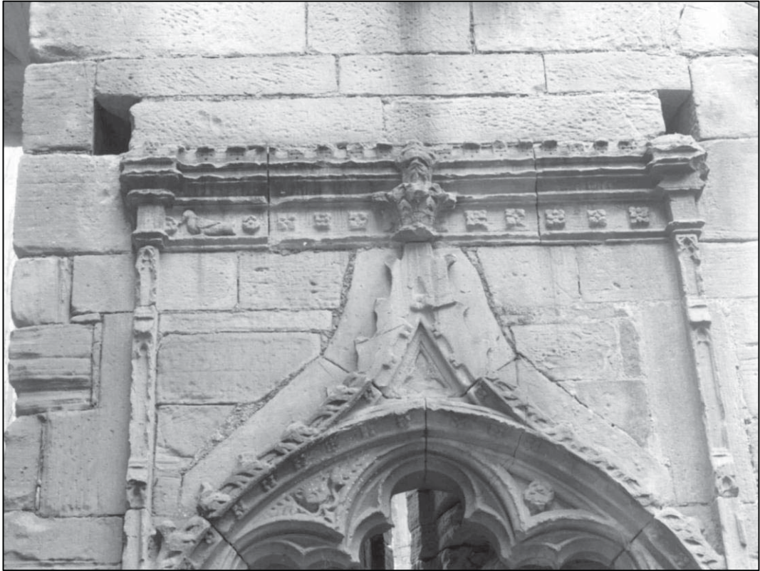
Plate 30: Detail of buffet in lower hall (elevation 22) (May 2000).
