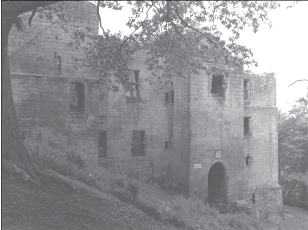
Plate 20: East side of castle (elevations 2 to 8), looking north-west (May 2000).
