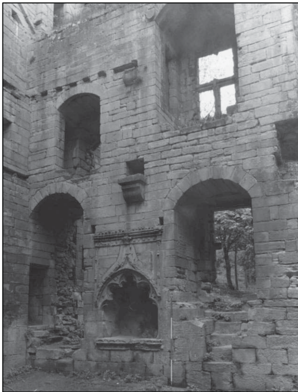
Plate 28: South end of west side of hall block (elevation 22) (May 2000).
