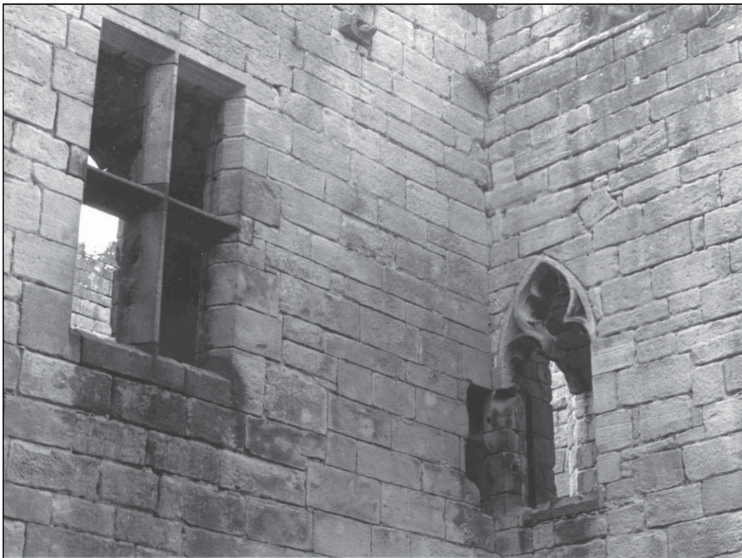
Plate 21: Junction of elevations 5 (W11) and 6 (W15), east side of castle (May 2000).
