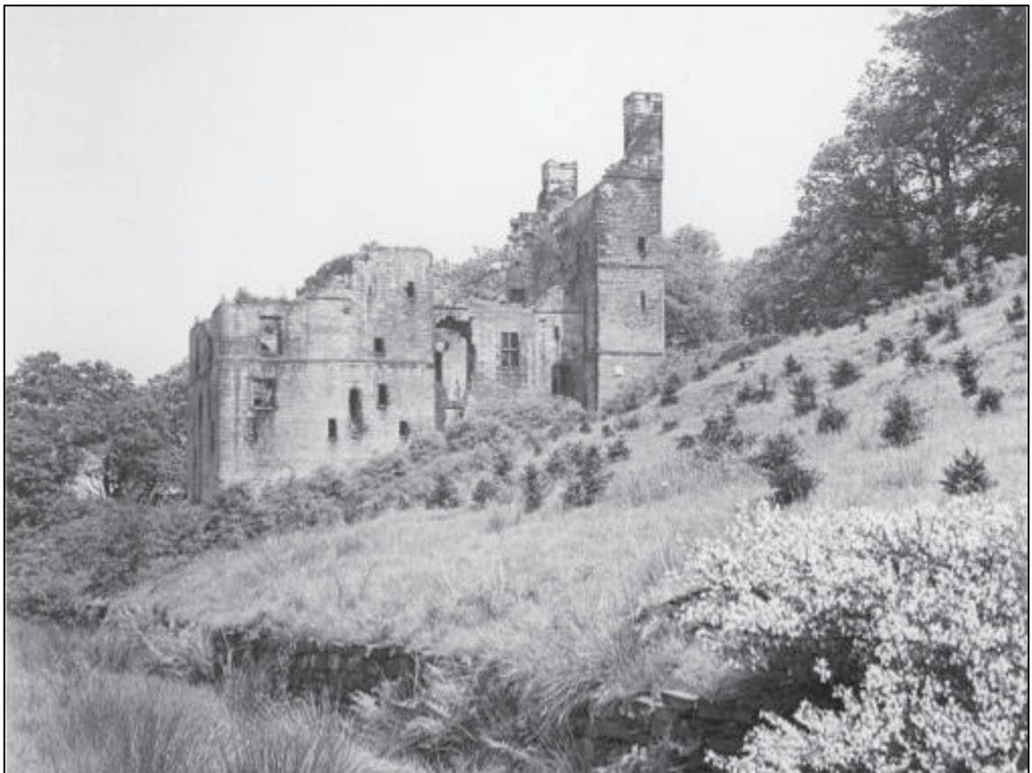
Plate 17: Undated photograph (c.1950s) of Harewood Castle, looking west (Harewood House Trust).
