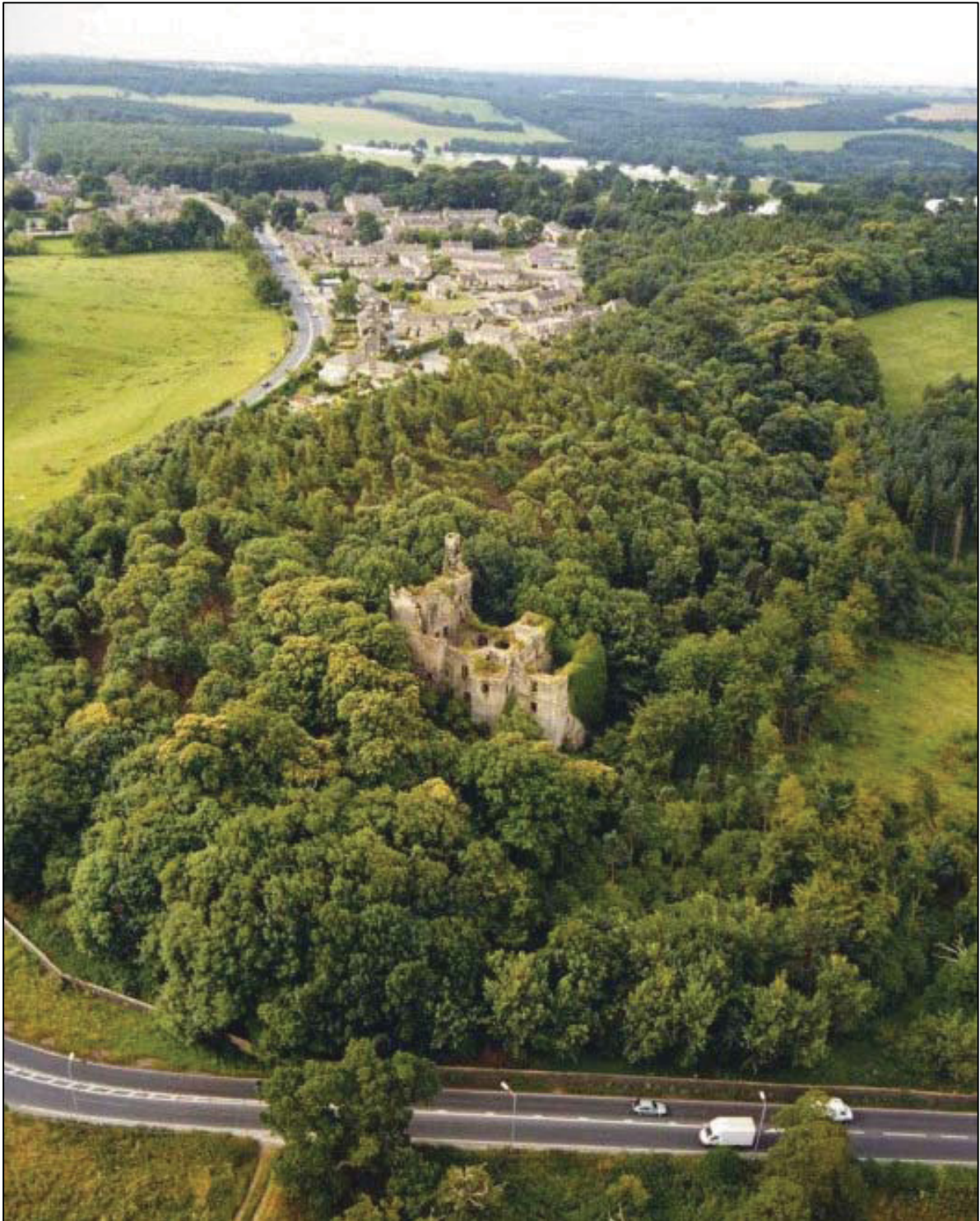
Plate 1: General view of Harewood Castle, looking south towards Bondgate (Harewood House Trust).
