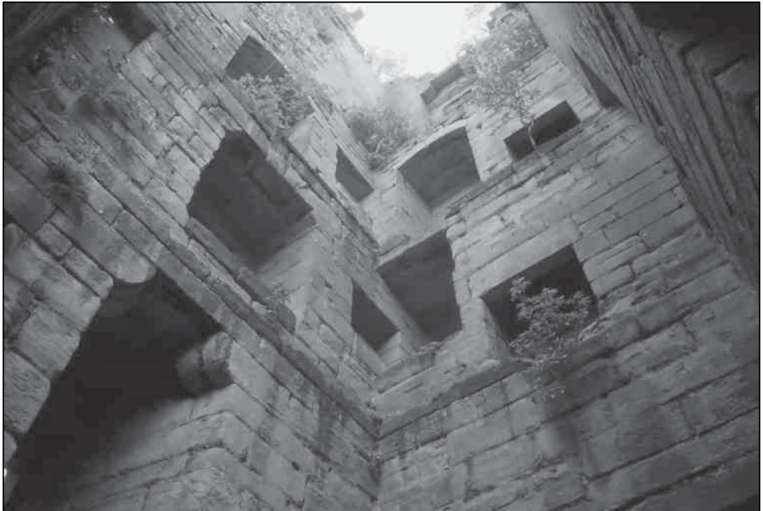
Plate 31: View looking up south-east tower (May 2004).
