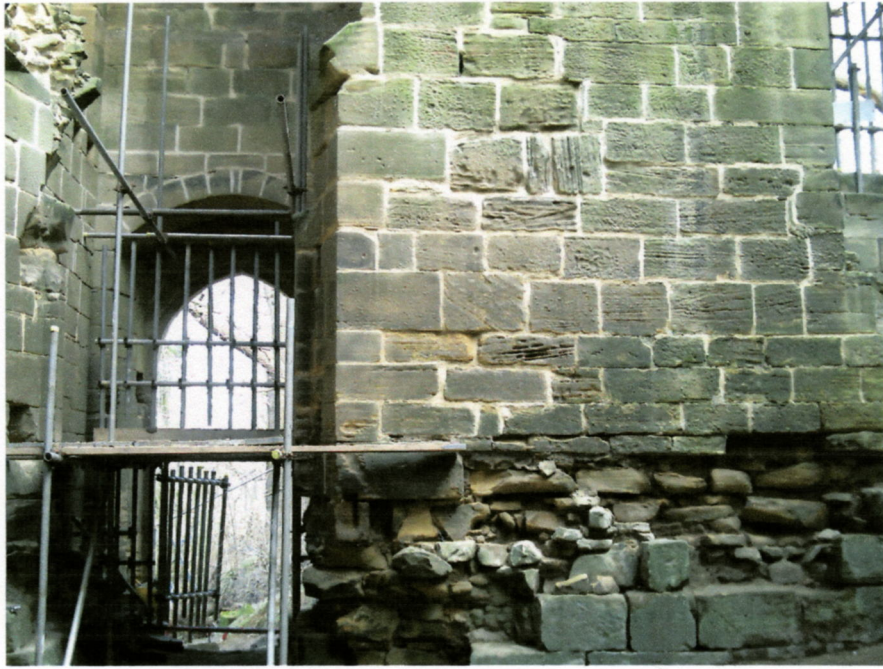
Figure 1. View towards main gate from central space. The use of plane bedded blocks on the corner contrasts with the blocks showing cross-bedding used in the rest of the wall.
