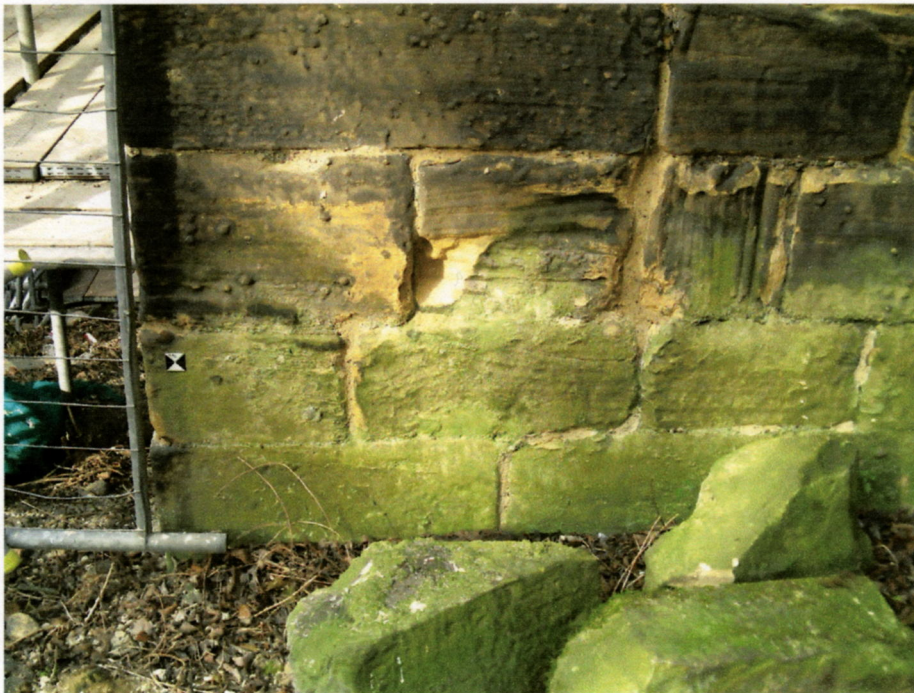
Figure 3. The single block on the exterior walls placed face-bedded. The block is spalling badly.
