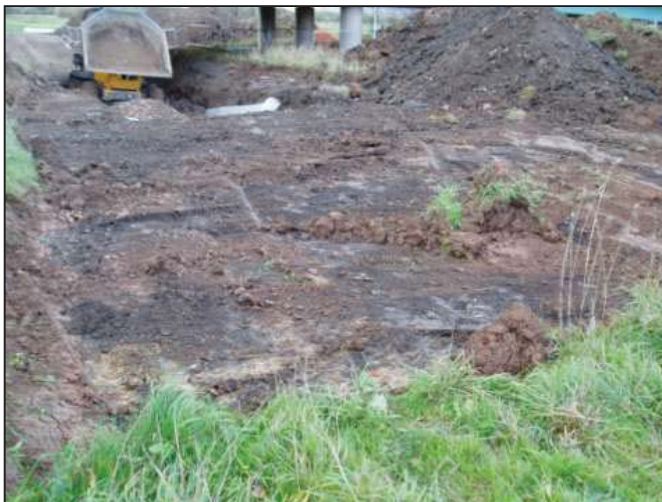
Plate 1: Excavation of Trench 4 Looking Southwest. No Scale.
