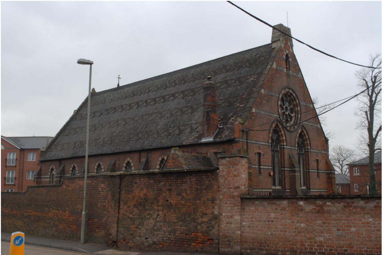
Plate 7 : The Old Chapel from the northeast
