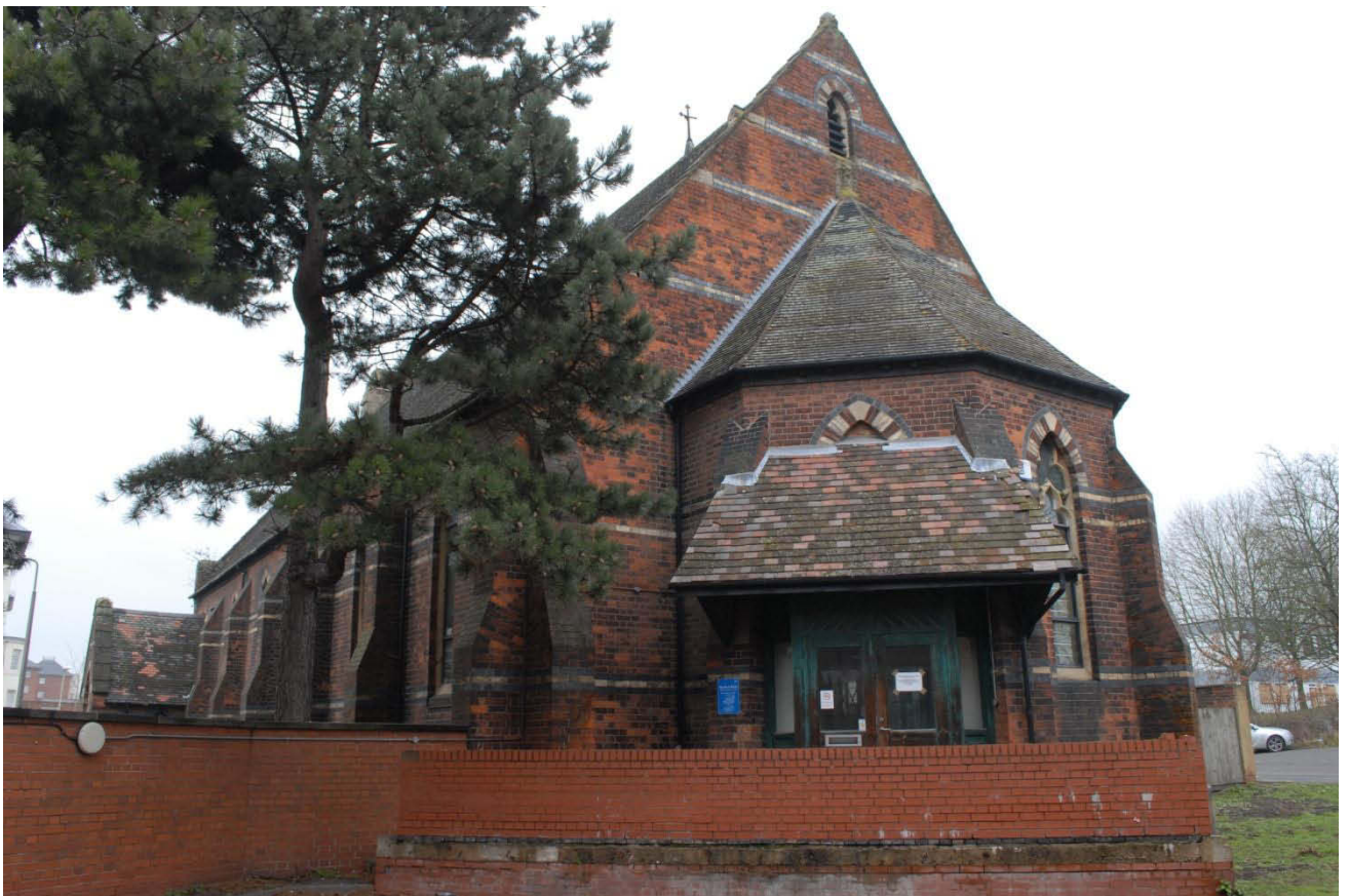
Plate 10 : The Old Chapel from the southwest
