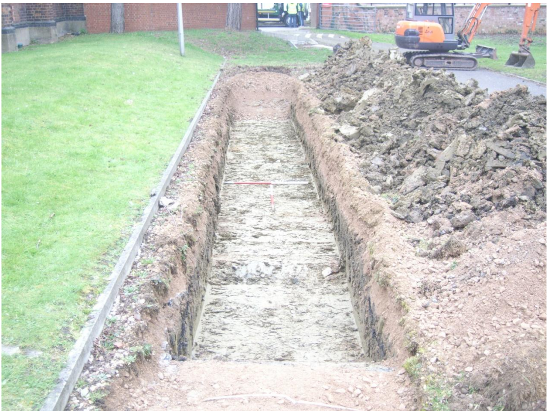
Plate 2 : Trench 1 looking south with electric cable in foreground (Scales 2 x 1m)
