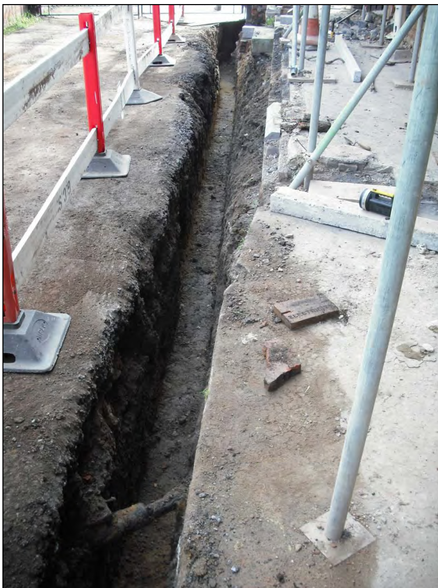
Plate 1: Trench 4 following excavation looking southwest (No scale).
