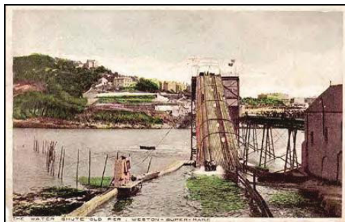
Old Pier Weston-super-Mare 1938 (Olney 2008)
