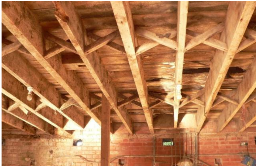
Alternating joists and herringbone strutting in north wing
