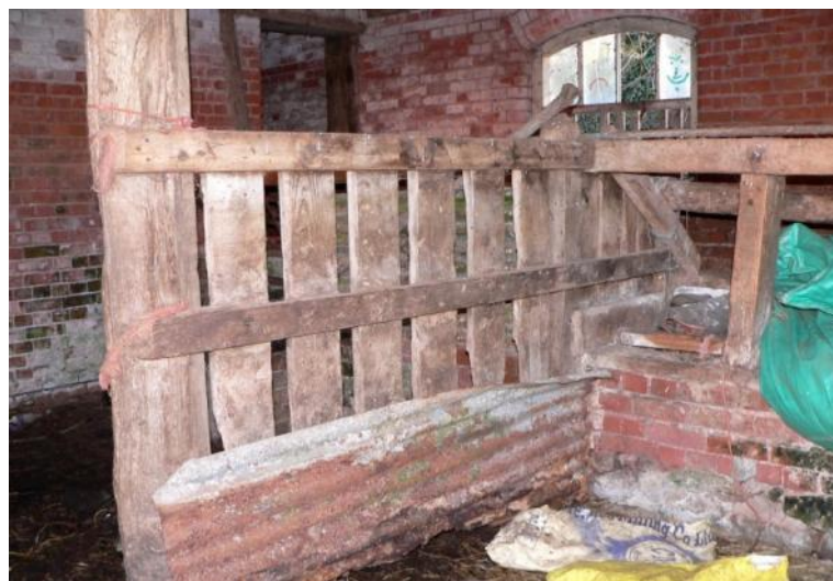
Stall division and feed trough, ground floor, south wing
