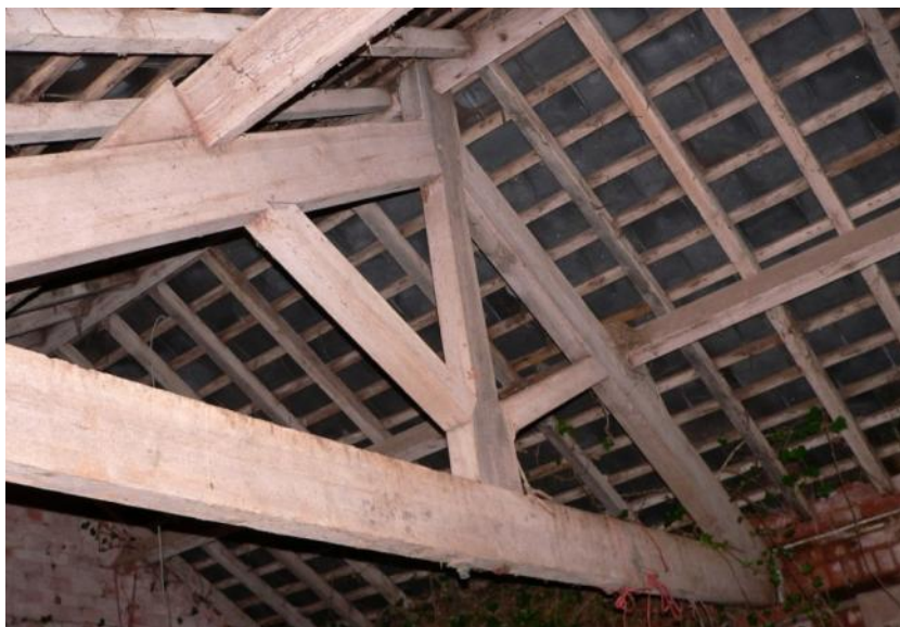
Roof truss and roof construction, west range
