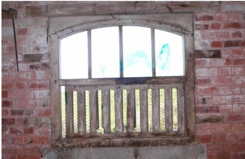
Detail of window and ventilator, west range
