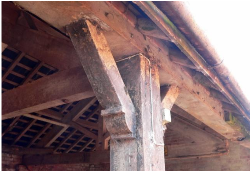
Detail of decorative bracing to head of linhay post
