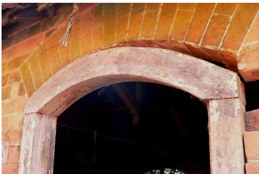
Detail of arched head of door frame
