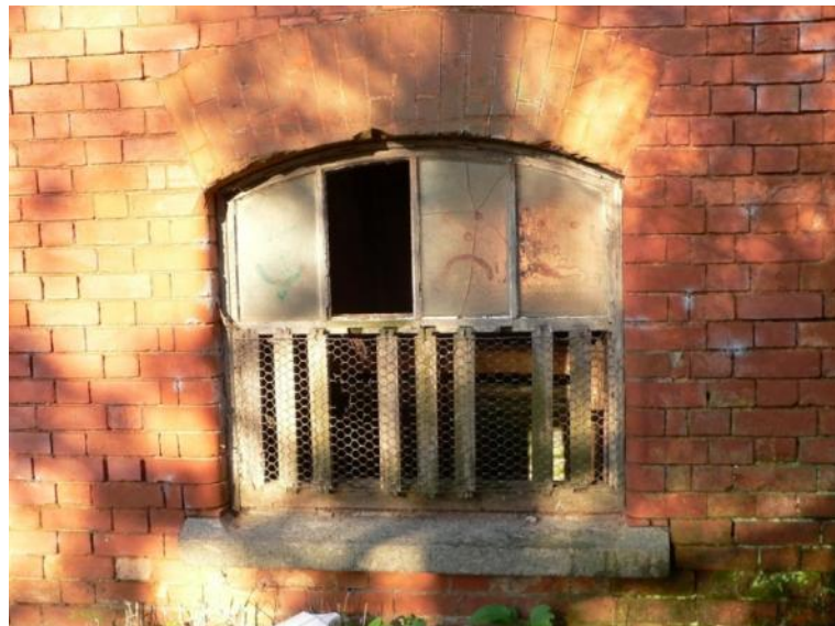
Ground floor window and sliding ventilator
