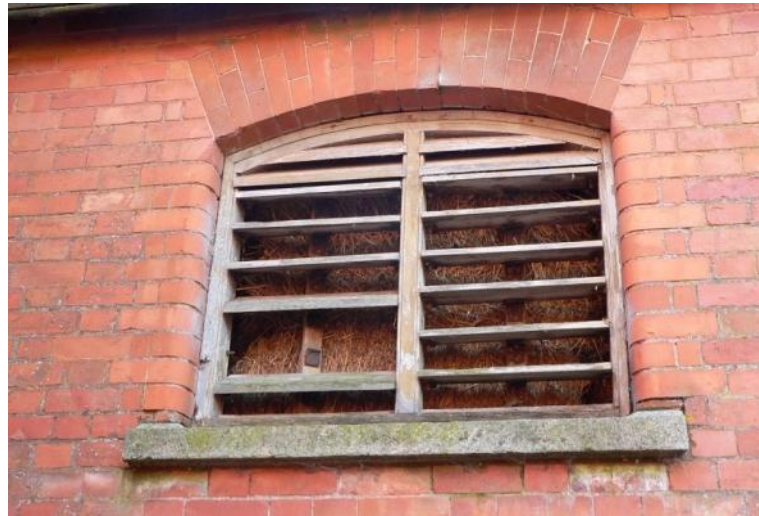
First floor louvred ventilator
