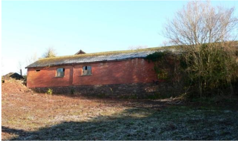
West elevation of west range, showing stone revetment below brickwork
