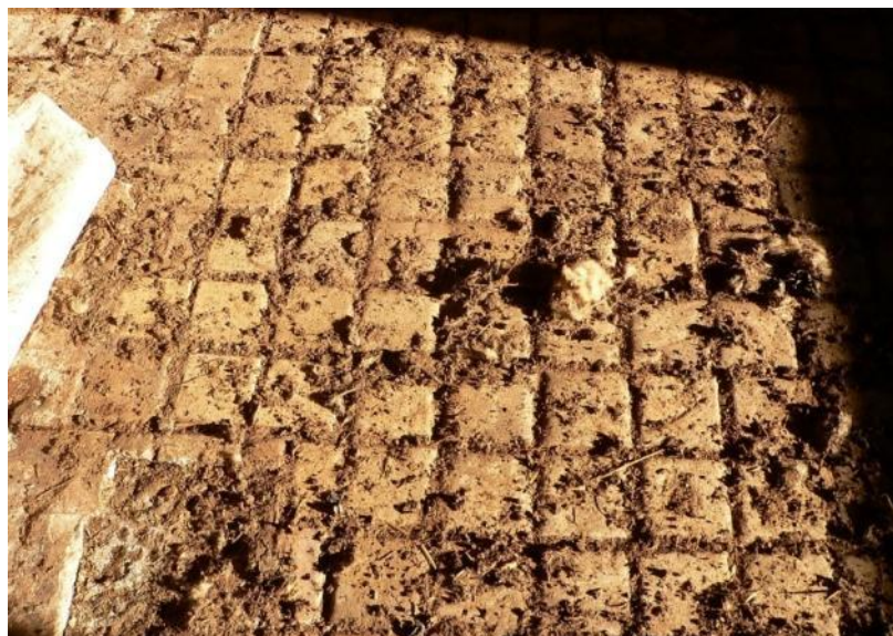
Stable paving bricks, ground floor, north wing
