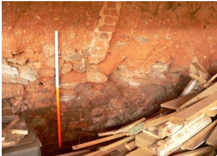
Rear wall, showing stone footing and eroded cob
