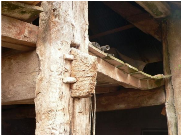
Wider front post and beam with through tenon and pegs at west end
