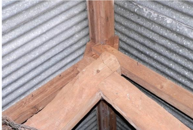
Apex junction of truss principals
