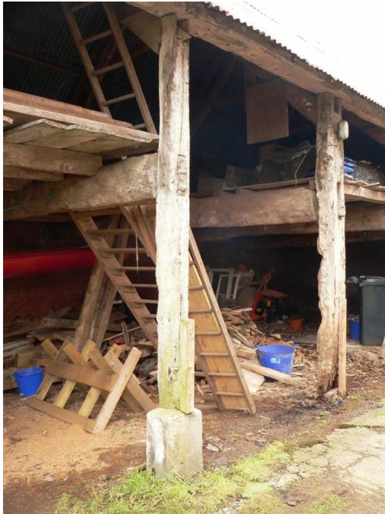
Bay 5, with concrete foot to front post
