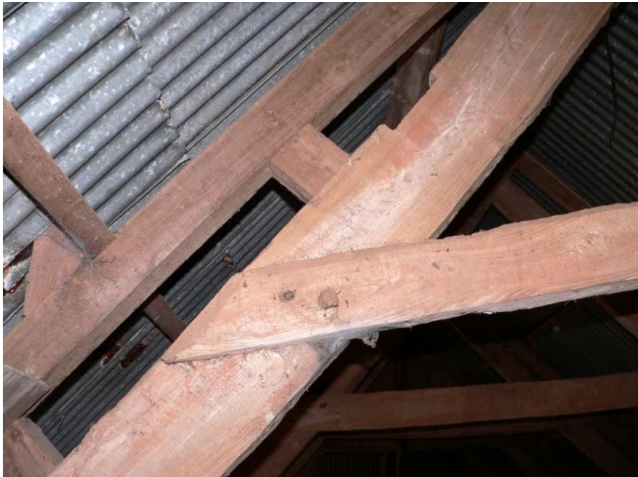
Detail of T6, showing collar/principal junction and former purlin trench
