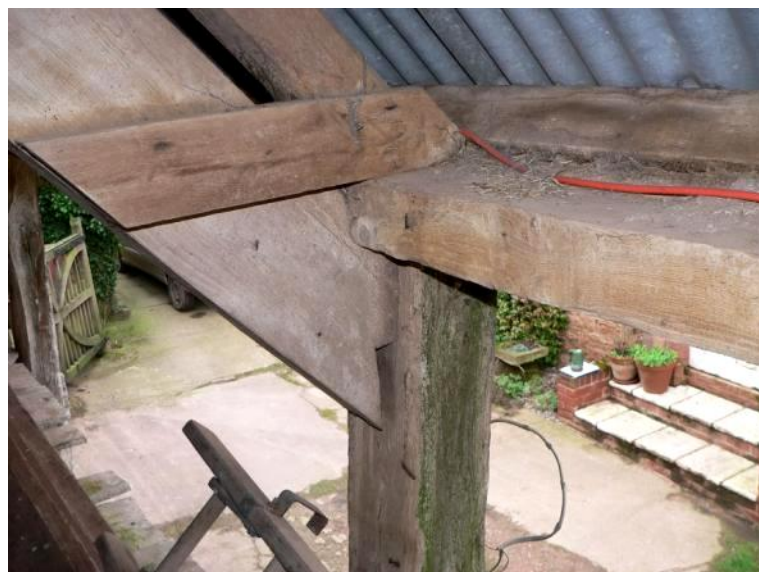
Front foot of principal tenoned into front post
