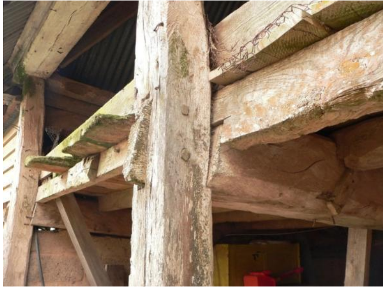
Front post and cross beam with pegged tenon at east end
