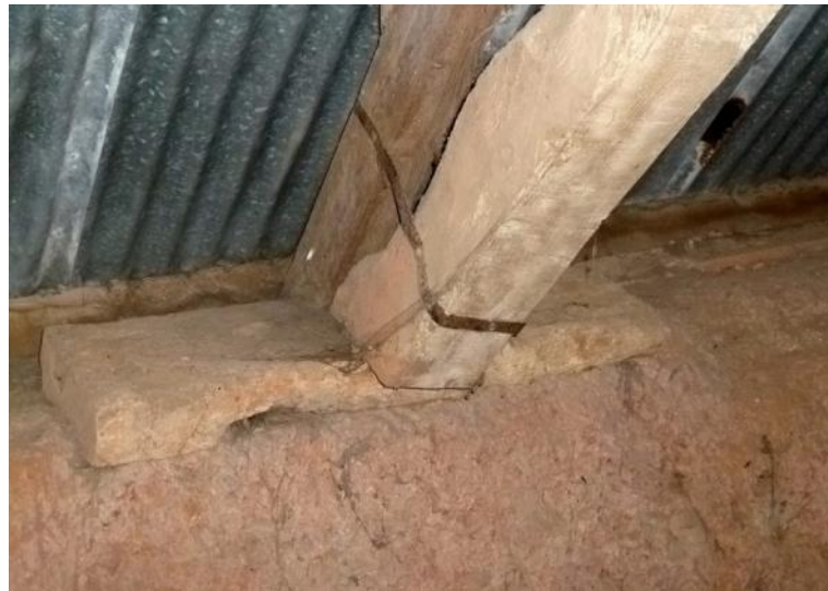
Foot of principal and timber plate on rear cob wall head
