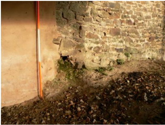
Bedrock exposed in rear wall of centre bay
