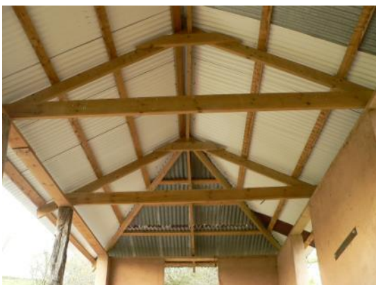
New roof structure, looking to west end
