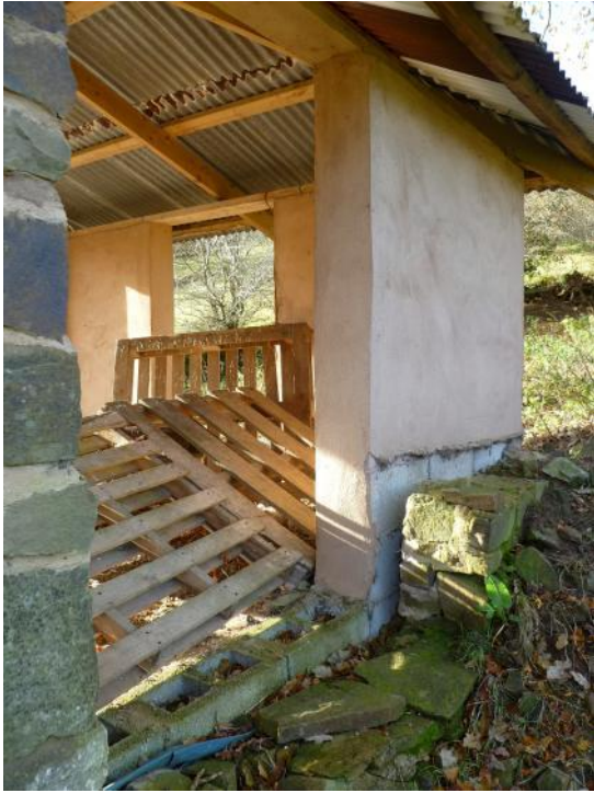
Doorway in north wall, bay 1 from west
