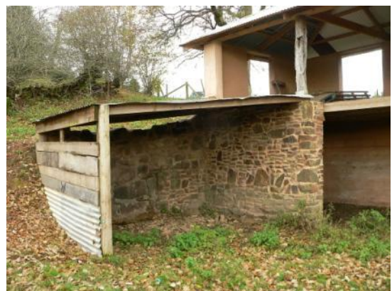
Lean-to extension, with rear (west) wall built into bank
