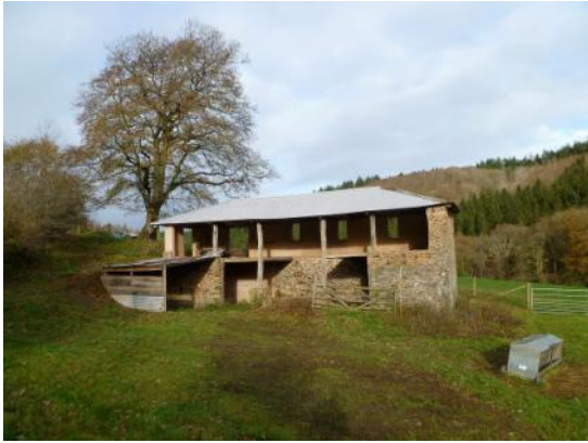
General view from the south
