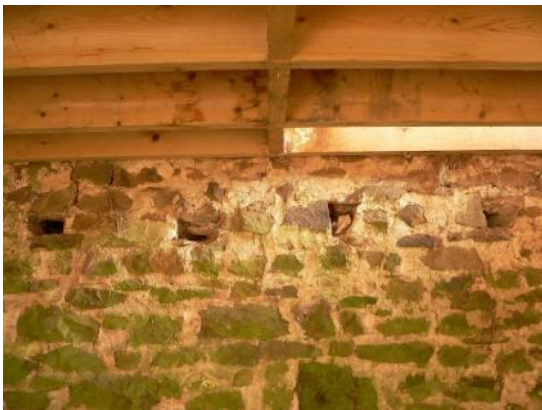
Joist sockets in east gable wall
