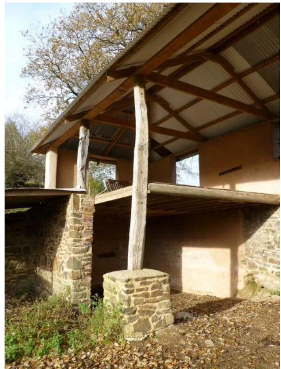
Centre bay, looking north-west, showing front posts and rendered concrete blockwork internal wall lining
