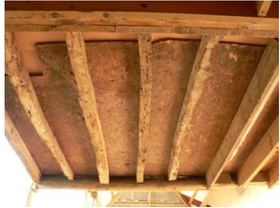
Reused floor joists in bay 4 from west
