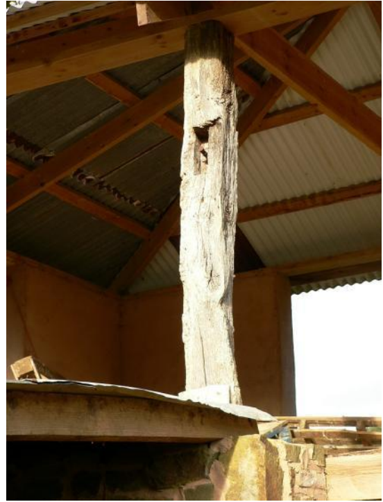
Re-used front post between bays 1 and 2
