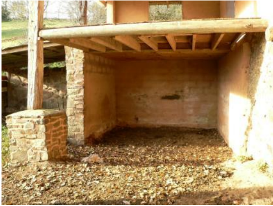
Ground floor interior, looking west
