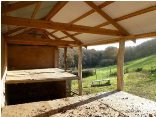
General view of first floor looking south-east
