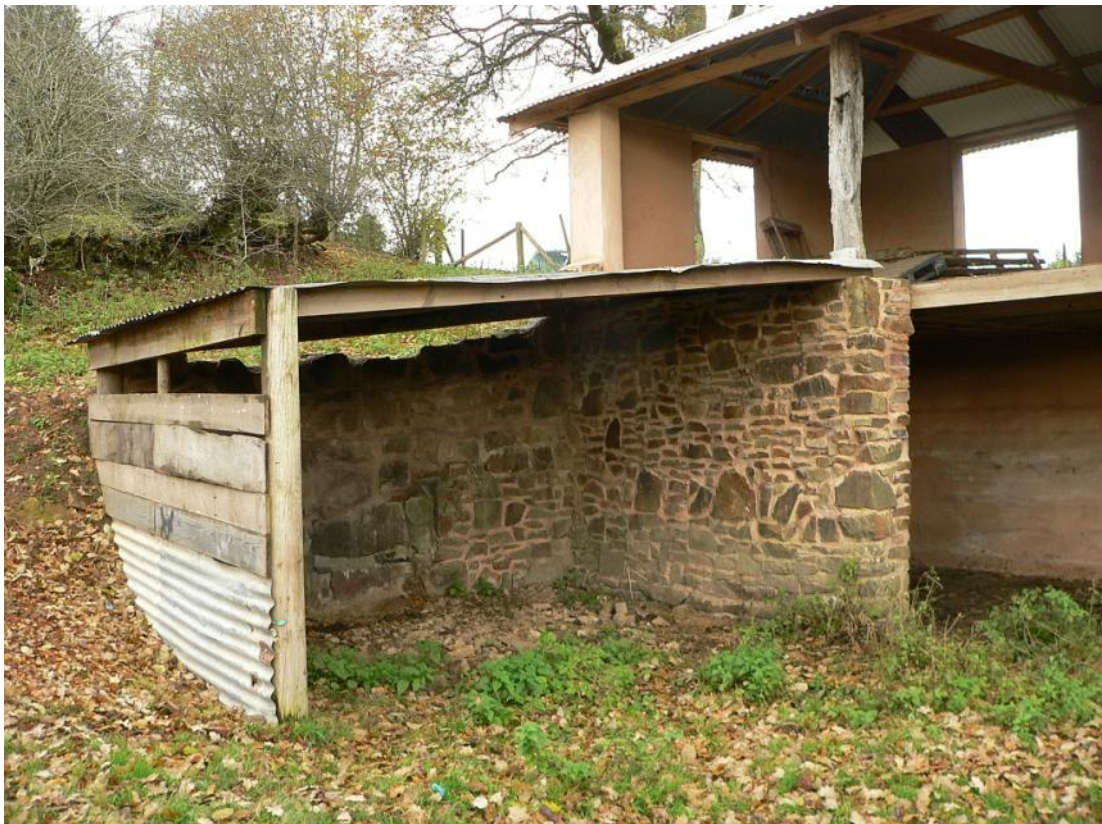
Lean-to extension at south-west end of linhay
