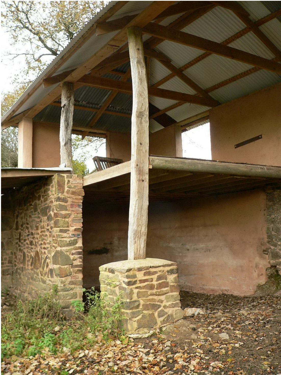
Linhay, looking north-west through centre bay, showing rebuilt and new stonework and rendered interior walls
