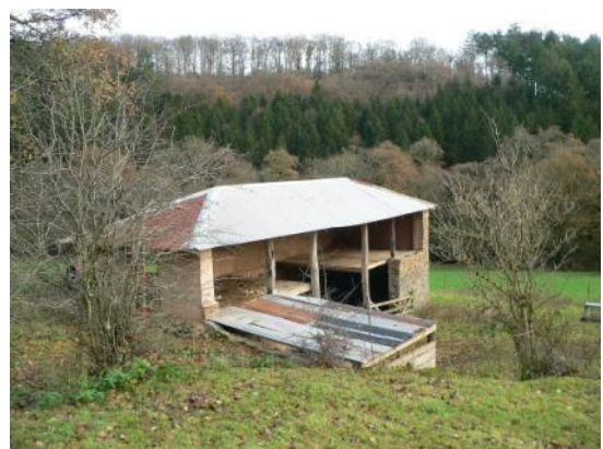
General view of linhay from rising ground to the south-west
