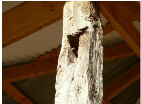
Detail of shoulder and mortice (upside down) on re-used front post
