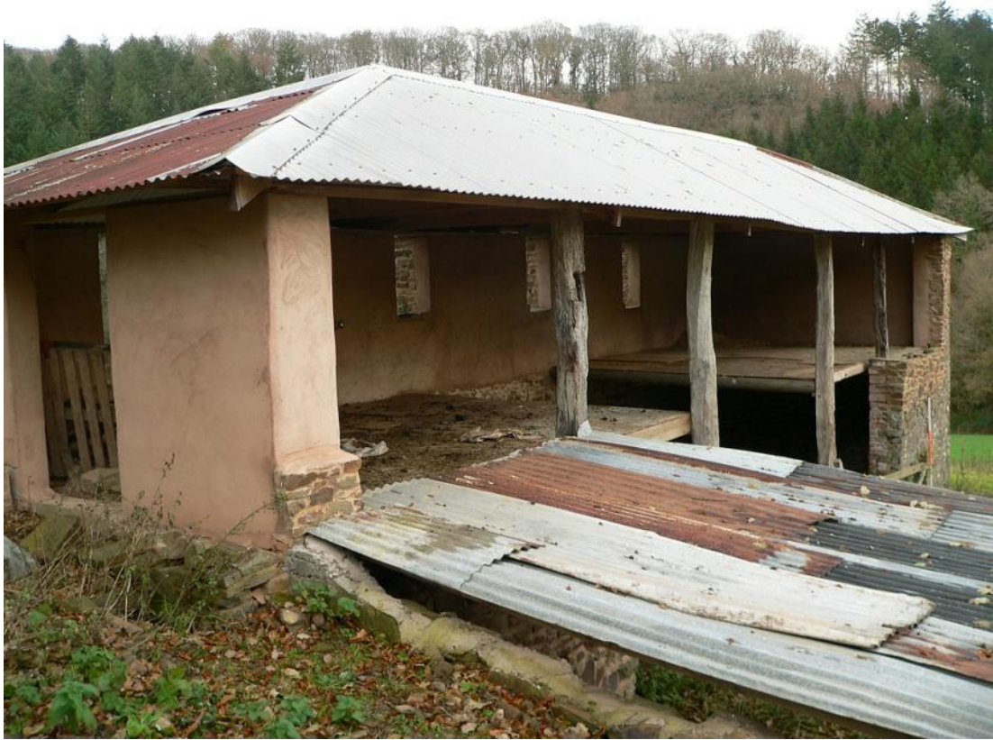
Linhay from rising ground to south-west, looking over lean-to roof
