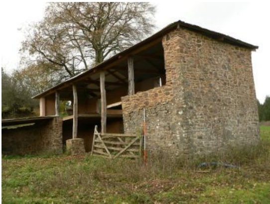
South front and east gable
