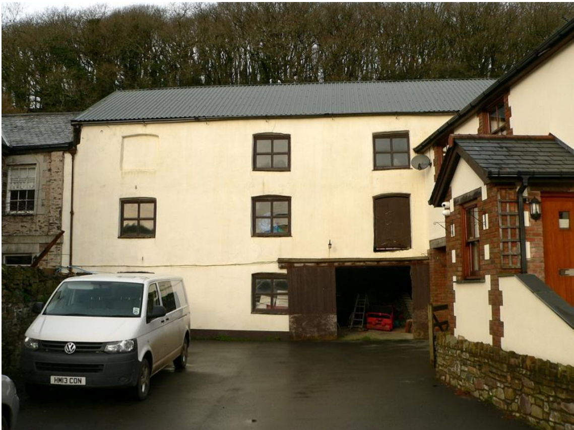
Heddon Mill: east elevation
