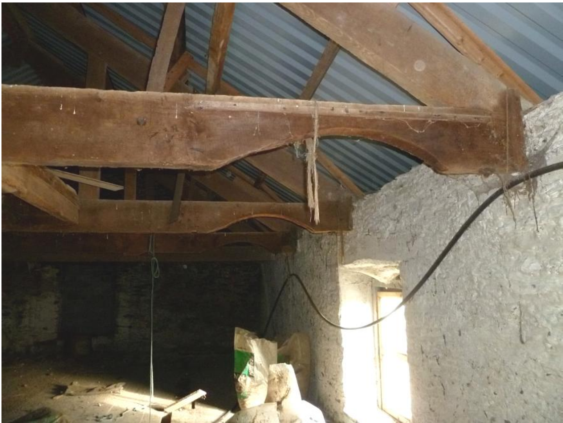
Cut-outs in roof truss tie beams, looking north-east
