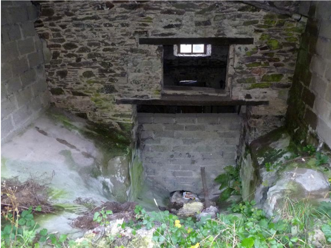
Intake pit on west side
