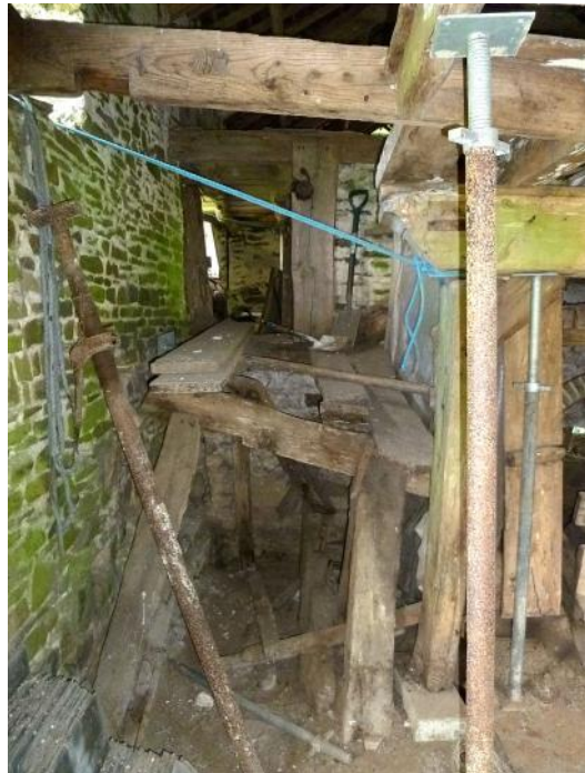
Remains of platform at east end of hurst, with ancillary drive support timbers beneath
