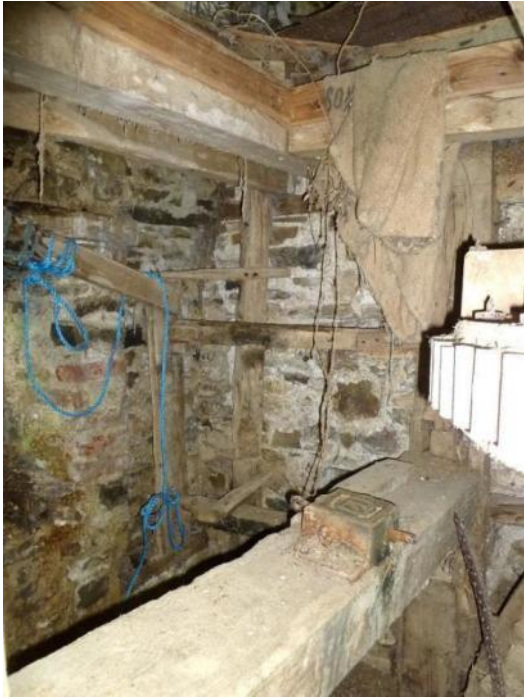
< Bridge tree and north-west corner under hurst in south mill
