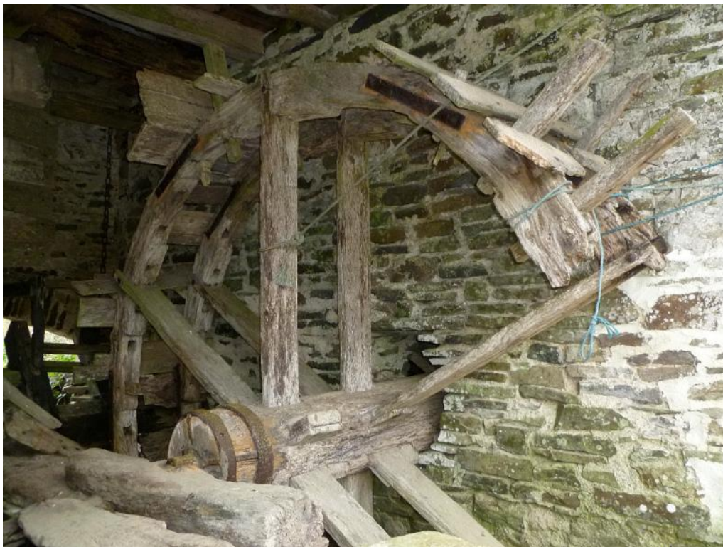
South waterwheel. Note the sawn off arm on the outer side
