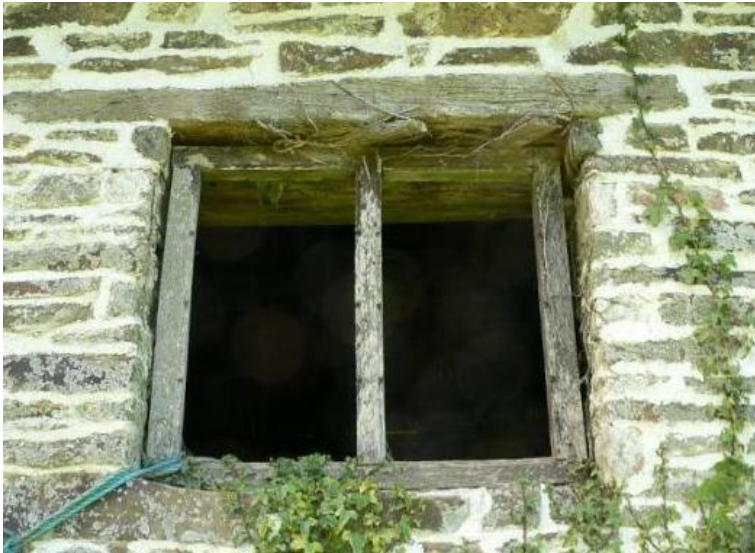
Timber-framed two light window, east elevation of north mill
