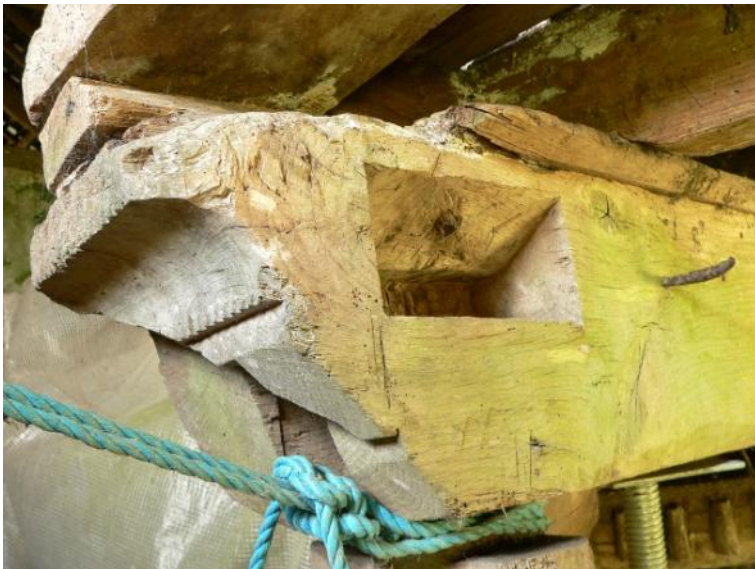
Moulded upstream end of hurst bressummer
