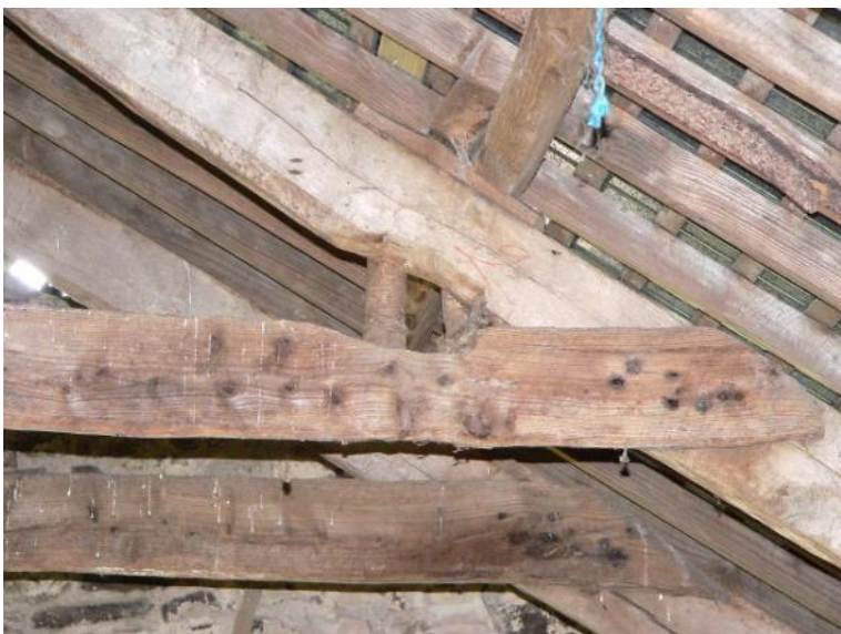
Detail of collar/principal joint, T5, with roundwood uprights for rope guide?
