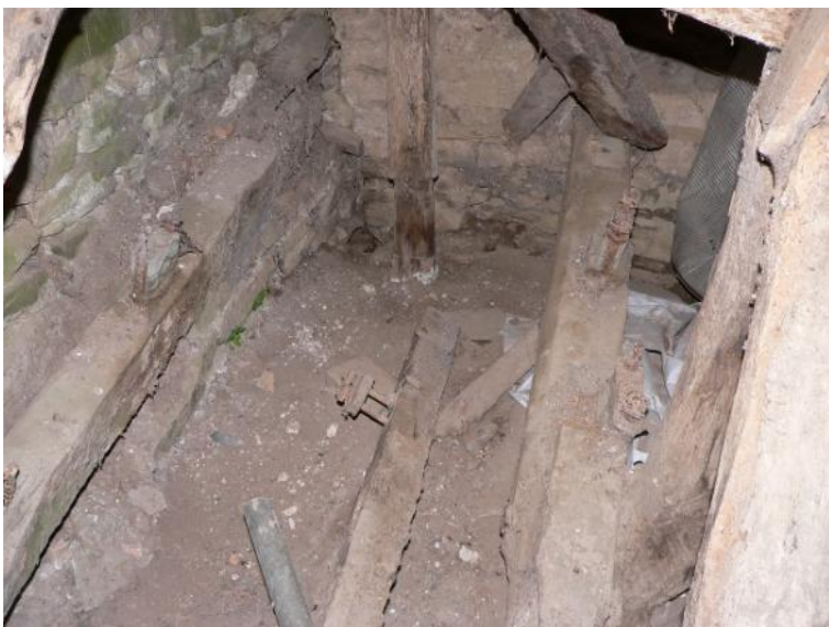
Ancillary drive support timbers with bearing against east wall
