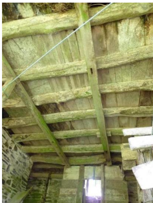
Floor support structure over central wheel chamber, looking east
