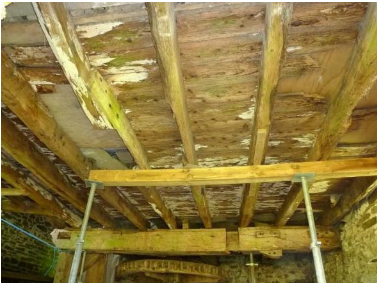
First floor joists, north mill, looking south to hurst frame
