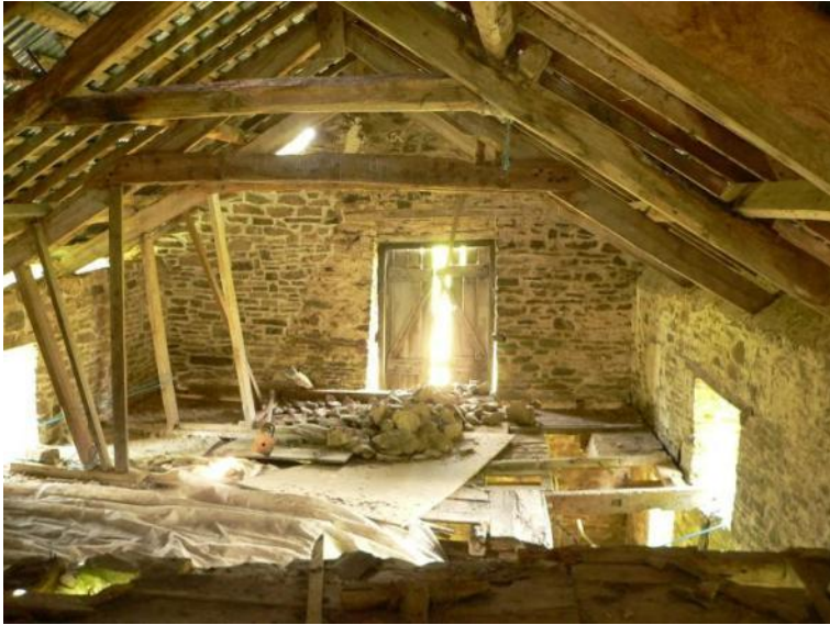
Roof structure and first floor of north mill
