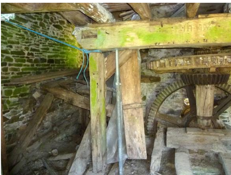
Position of raised platform at east end of hurst, north mill
