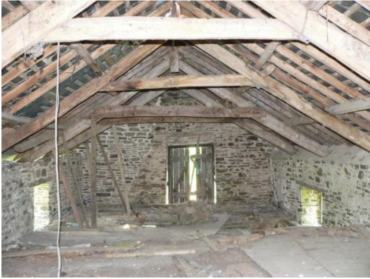
Roof structure, looking north
