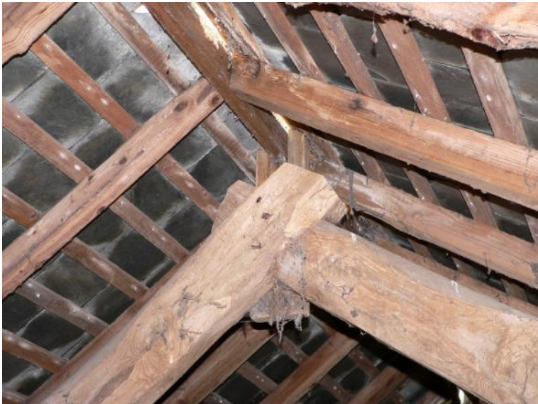
Detail of truss apex
