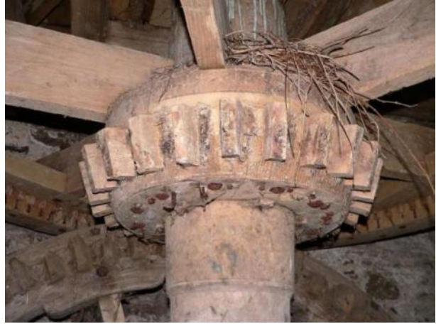
Detail of wallower, south mill
