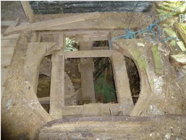
Millstone emplacement in hurst floor, south mill
