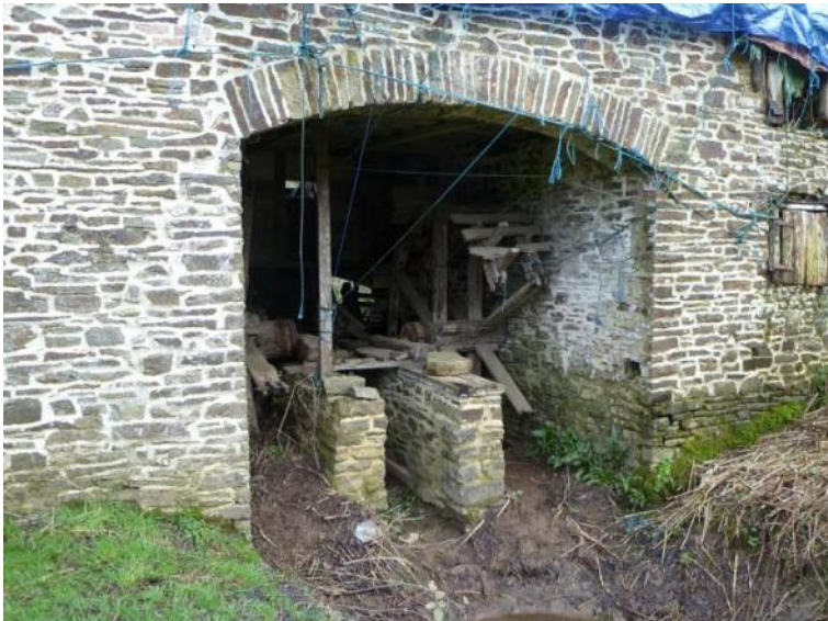
West end of wheel chamber and tailrace channel
