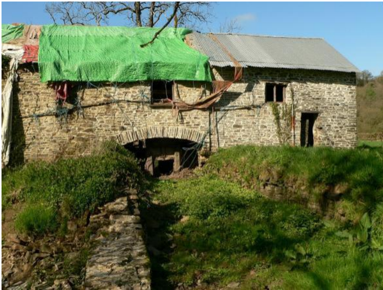
Headrace with wall to spillway on right
