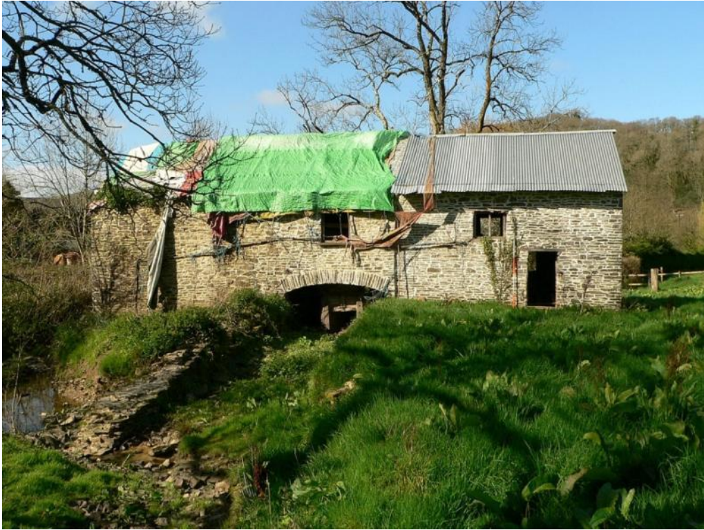
East elevation, with stone revetted leat and spillway to left
