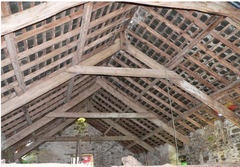
Roof, general view showing construction, looking to north
