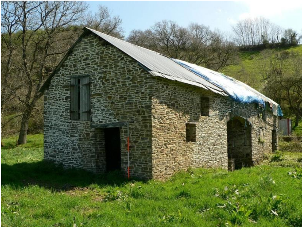
North gable and west elevation, from the north west
