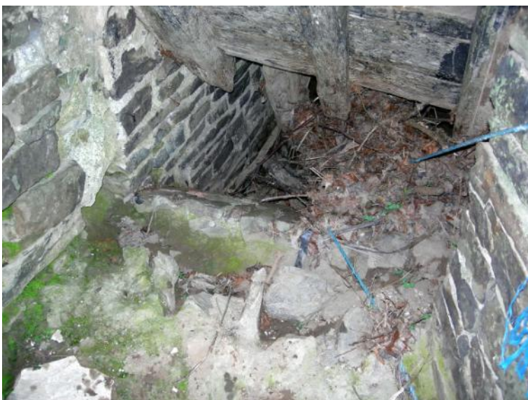
Displaced penstock to south waterwheel, showing edge of curved stone breastwork
