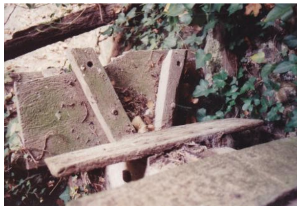
Remains of north waterwheel and detail of V-shaped start and float, July 1989
