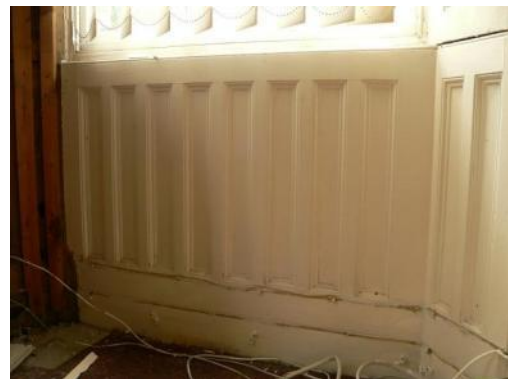
Detail of fielded panelling under window
