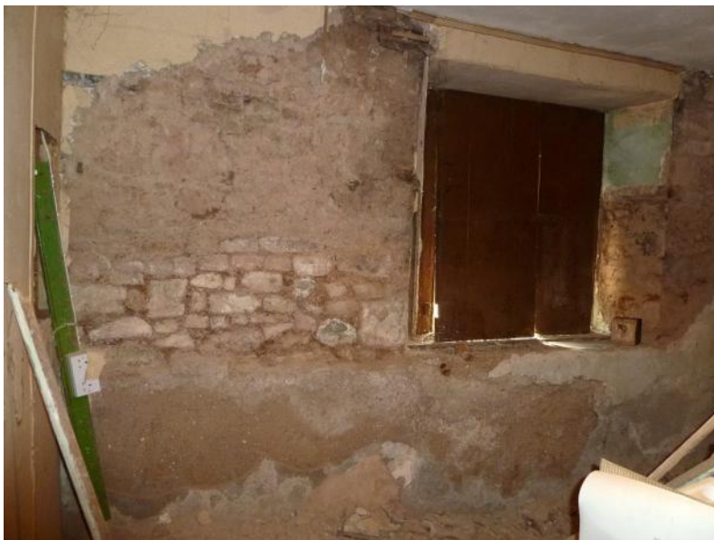
South room, interior of south wall showing exposed cob and masonry and shuttered window
