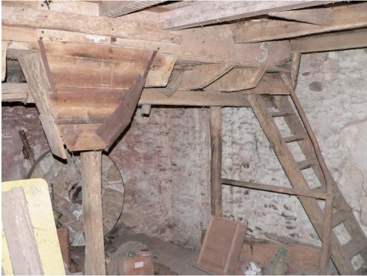
South-west corner of first floor, with steps up to second floor
