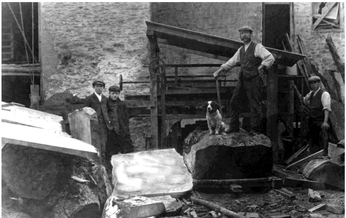
Figure 7: The sawmill outside of Manor Mill, c.1910 (from Jones & Hamilton 2010, 311, courtesy of Brian Murless). This appears to be a horizontal reciprocating saw.
