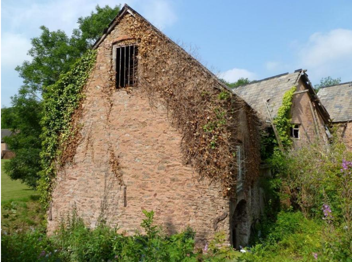
South-east gable end of workshop, from east
