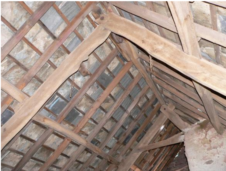
Mill roof, looking south-west to roof over kiln extension
