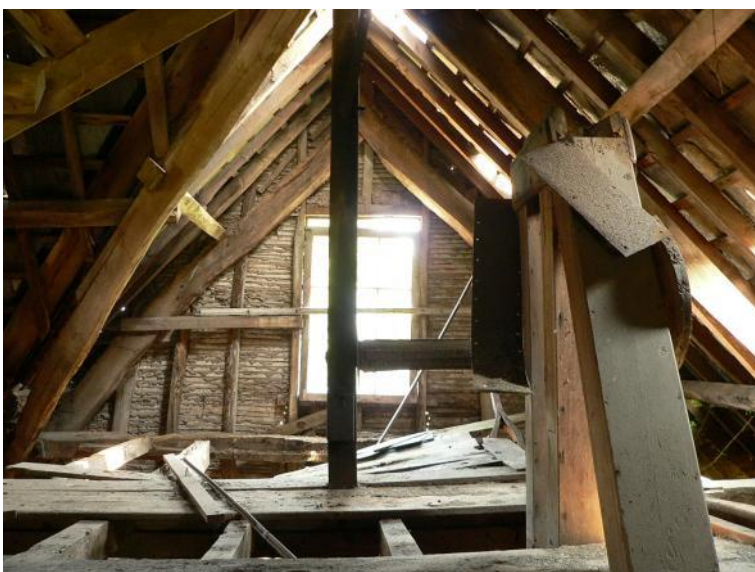
Loft gallery, looking to north-east, with stud and lath gable infill
