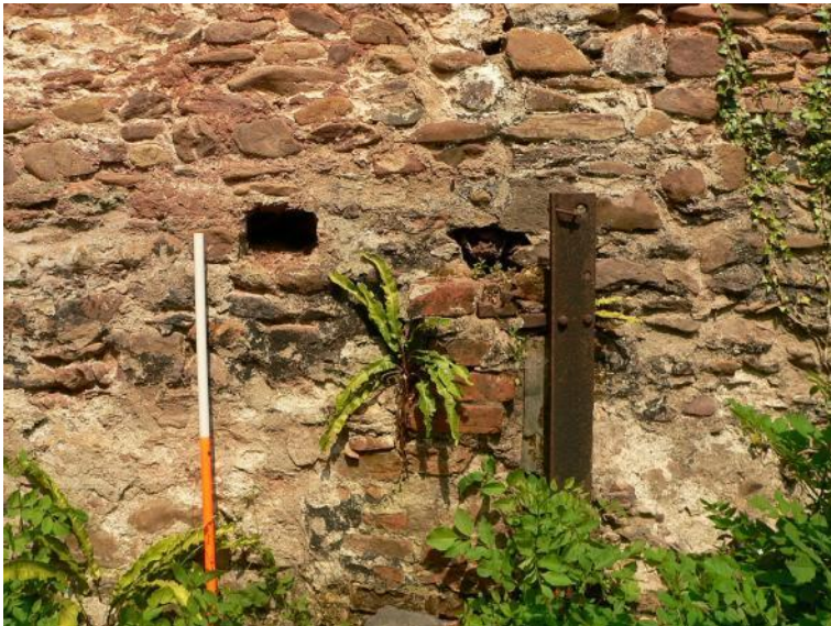
Brick pier at upstream end of former waterwheel pit
