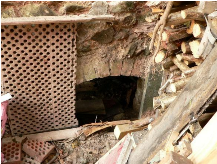
Arched opening to cog pit with fragments of kiln floor tile on left
