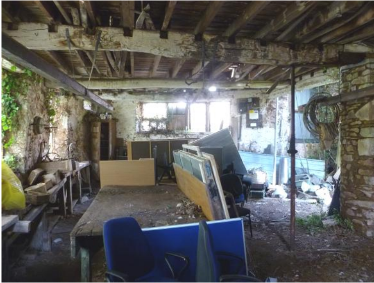
Workshop, ground floor, looking north-west
