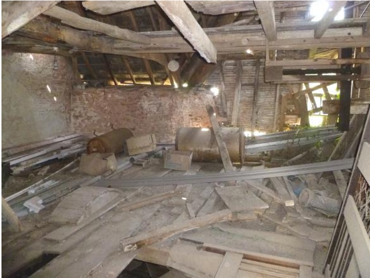
Loft floor of mill, looking north-east
