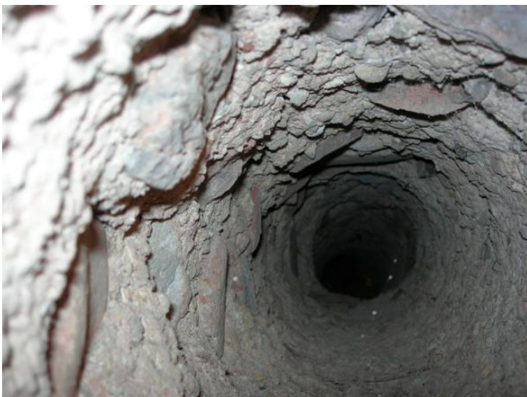
Kiln flue within thickness of wall, looking upwards
