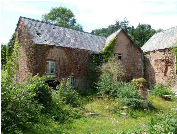
Workshop building from the railway embankment to the south-east
