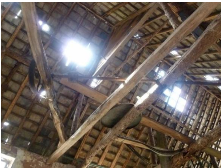
Roof of workshop, with skewed layshaft on principal beams
