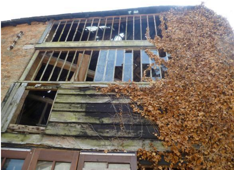
North-west gable windows to upper level of workshop
