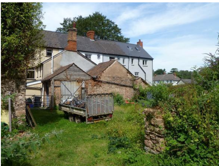
Site of former building adjoining rear and north-east end of mill
