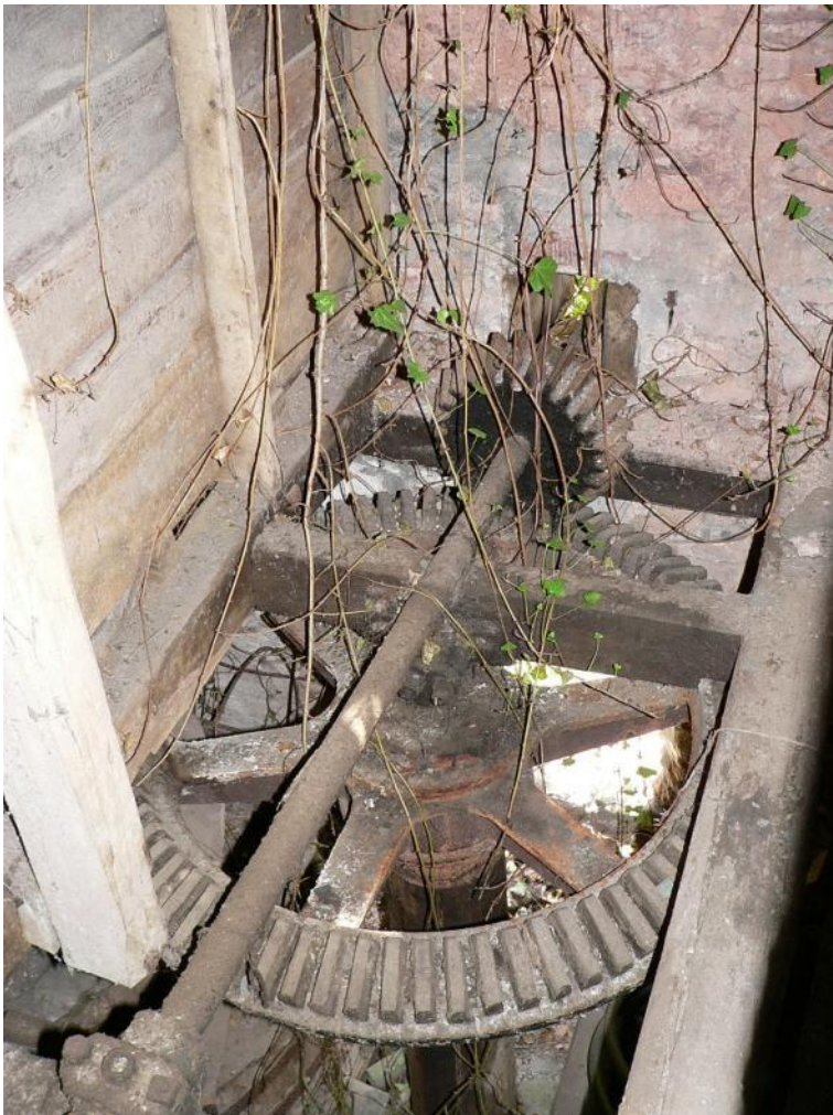
Crown wheel at top of upright shaft, with pinion on the far side, on layshaft extending through the pit wall and back into the mill
