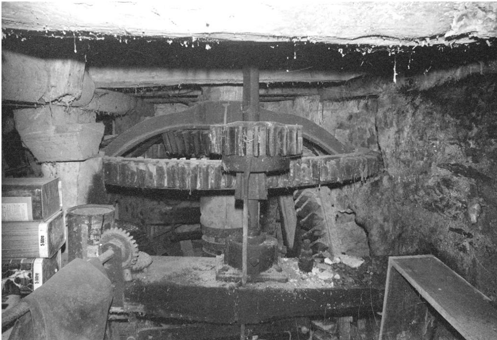
Figure 9: The drive to the upstream millstones, 1977 (D.W. Warren)
