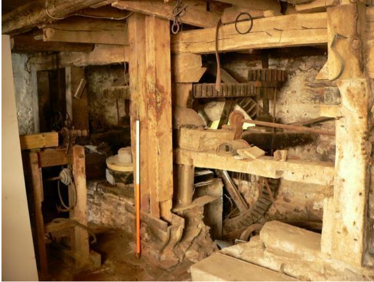
Mill ground floor: hurst and primary drive, looking east
