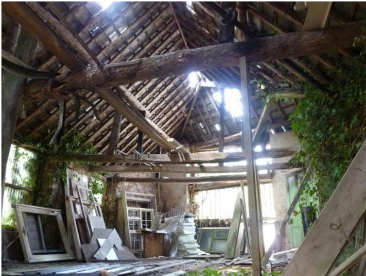
Workshop, first floor, looking north-west
