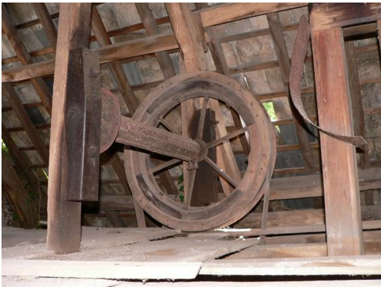
Sack hoist drive wheel and chain drum, with elevator to right
