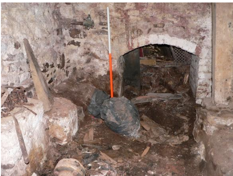
Upstream end of cog pit, with arch to lower level of former kiln
