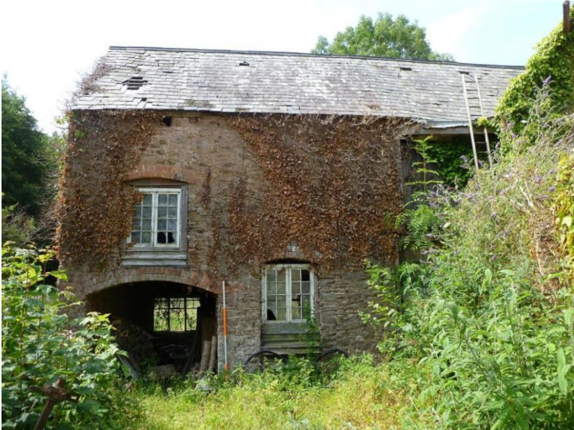
North-east elevation of workshop
