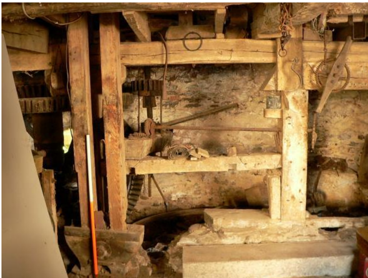
Hurst, bridging and tentering gear to upstream millstones
