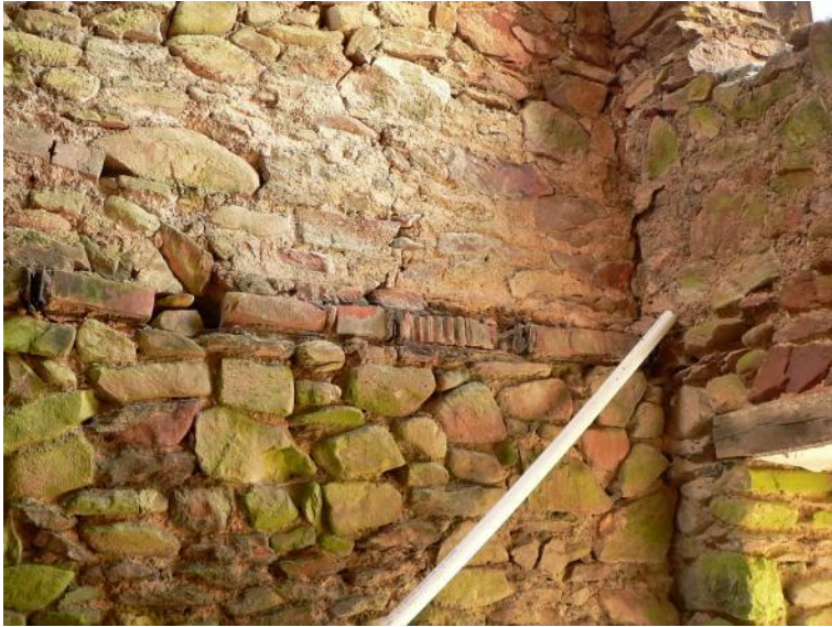
Remains of kiln floor tiles built into wall
