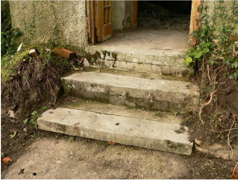
Lias slab front steps up to porch door
