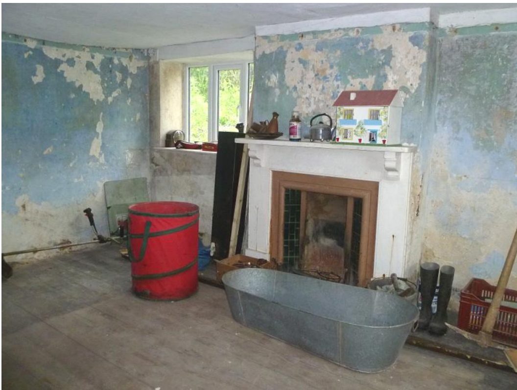
Ground floor, north room, showing fireplace surround and suspended timber floor
