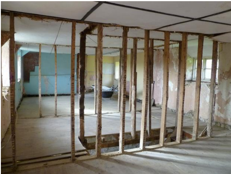
Stud partitions at head of stairway during demolition
