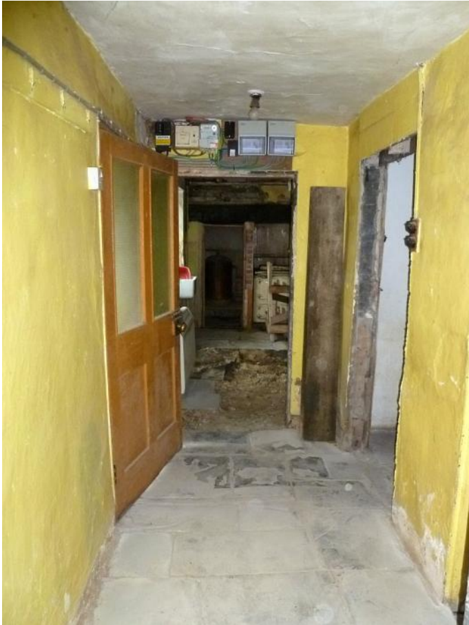
Ground floor passageway, looking south
