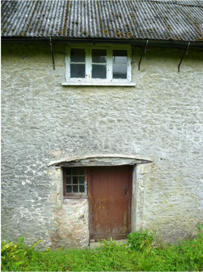
West elevation: back door (to former dairy) and timber-framed window to landing
