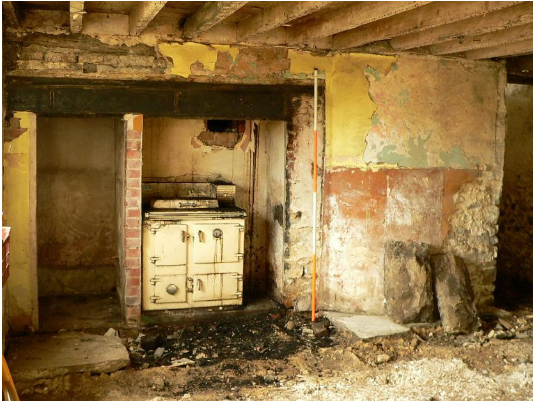
Ground floor, south end. Fireplace wall in former kitchen. Note remains of lias stone slab flooring
