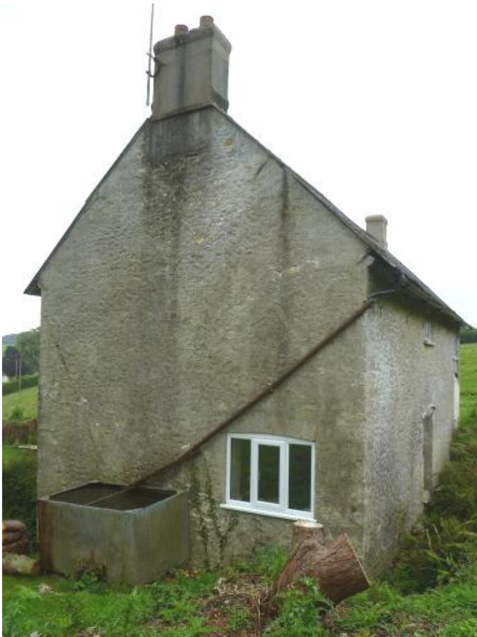
North gable end, looking along rear (west) of house
