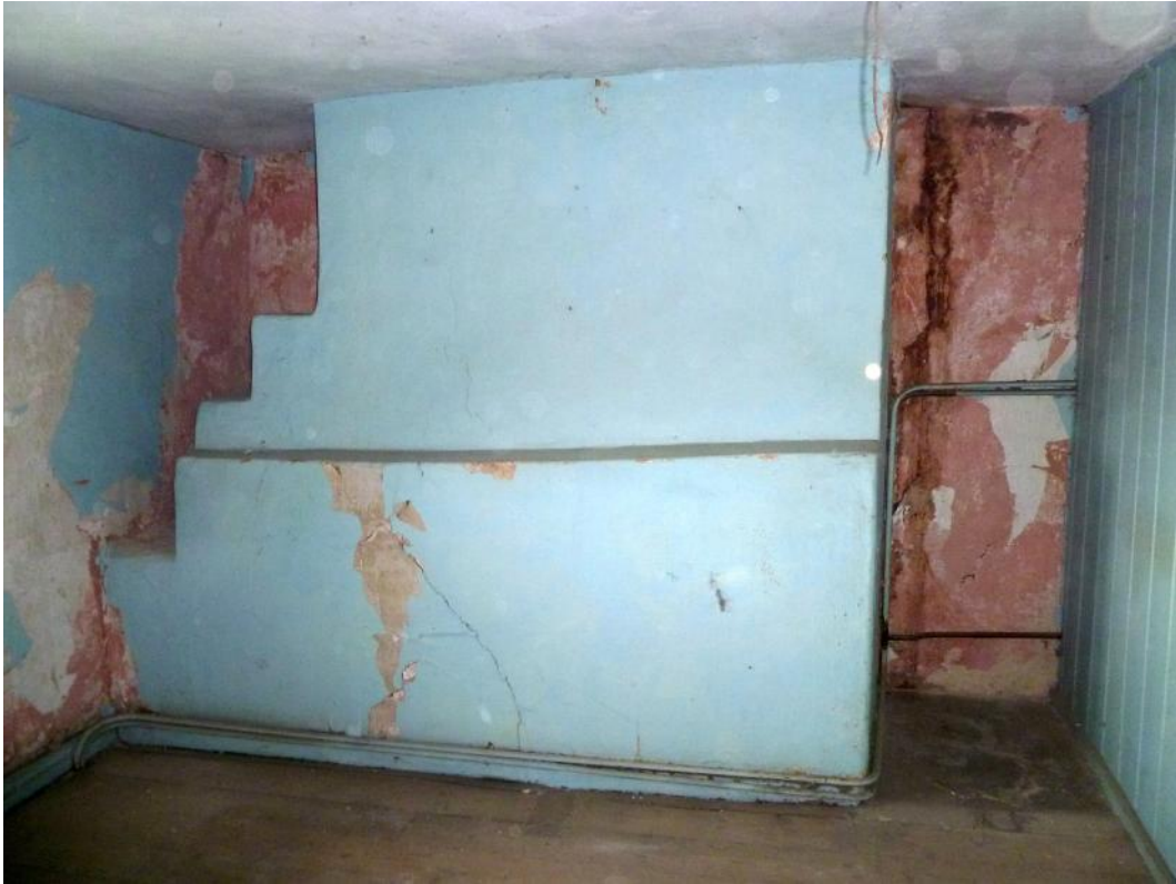
First floor, south room chimney breast, with bathroom partition on right
