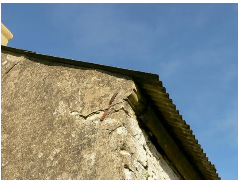
Moulded stone kneeler on south-east corner of south gable
