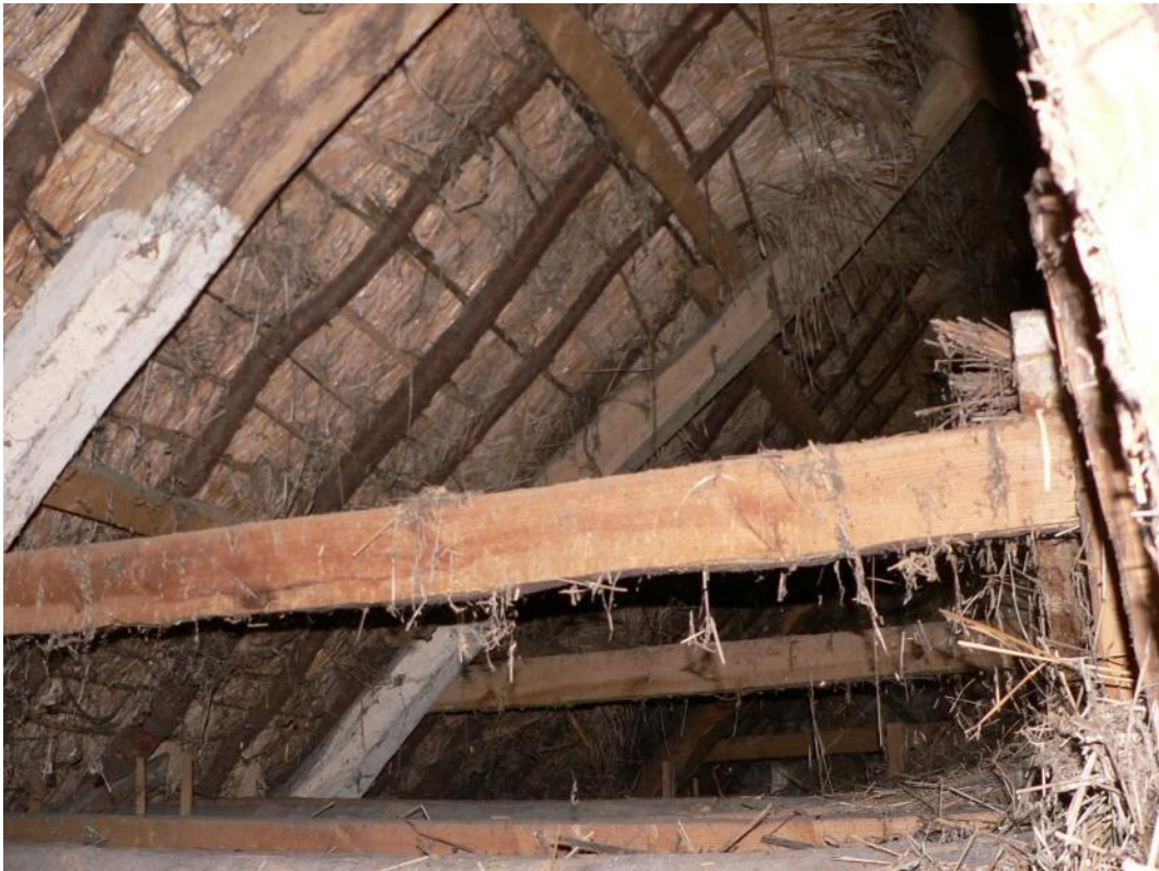
Roof structure, looking north from above south room
