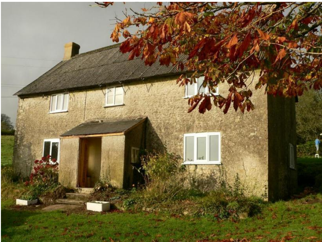
East elevation, from north-east
