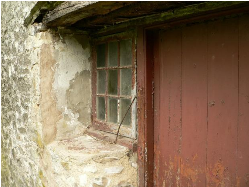
Back door and window to former dairy
