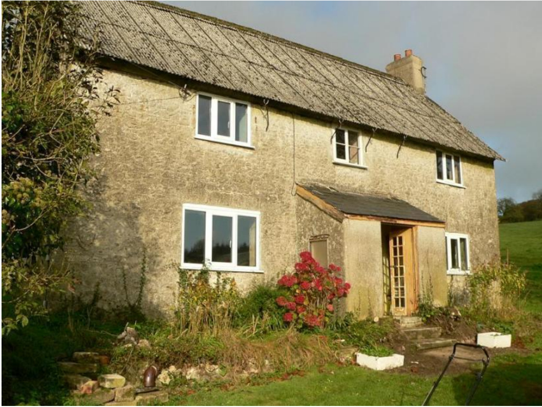
East elevation, from south-east
