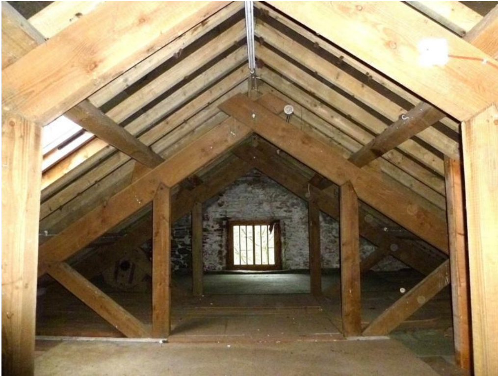
Reconstructed roof, looking east
