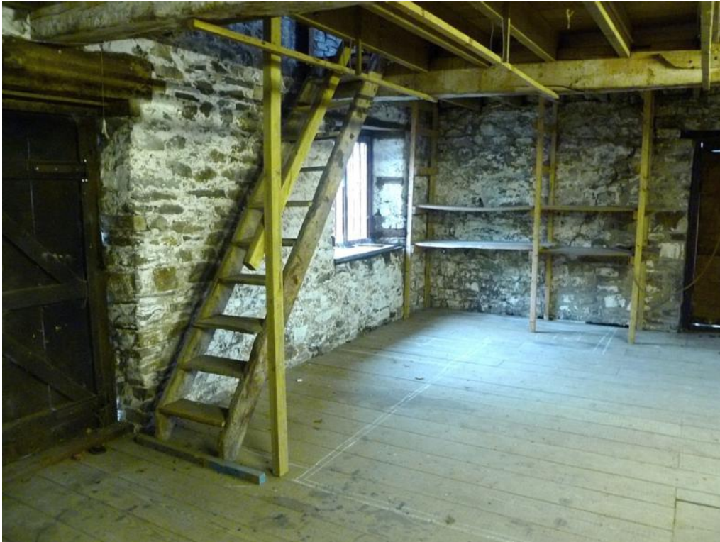
First floor, looking south west, with steps up to second floor
