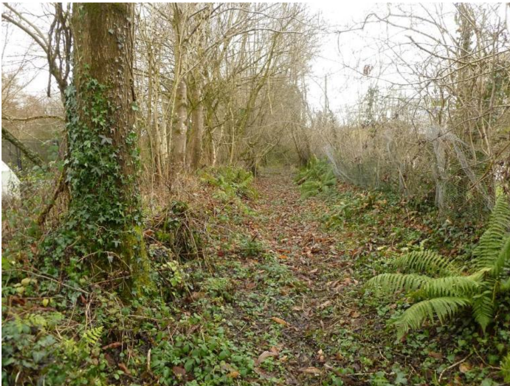
Silted section of leat to east of mill
