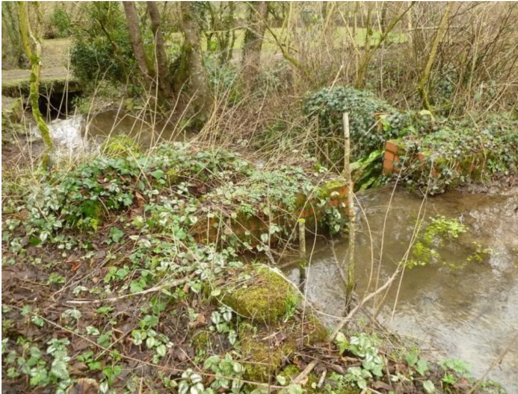
Leat diversion at spillway, with blocking to foreground
