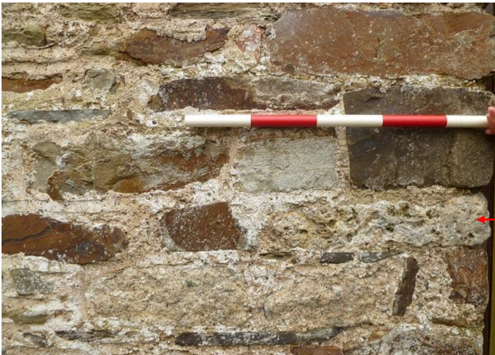
French burr millstone fragment built into west gable (half metre scale)
