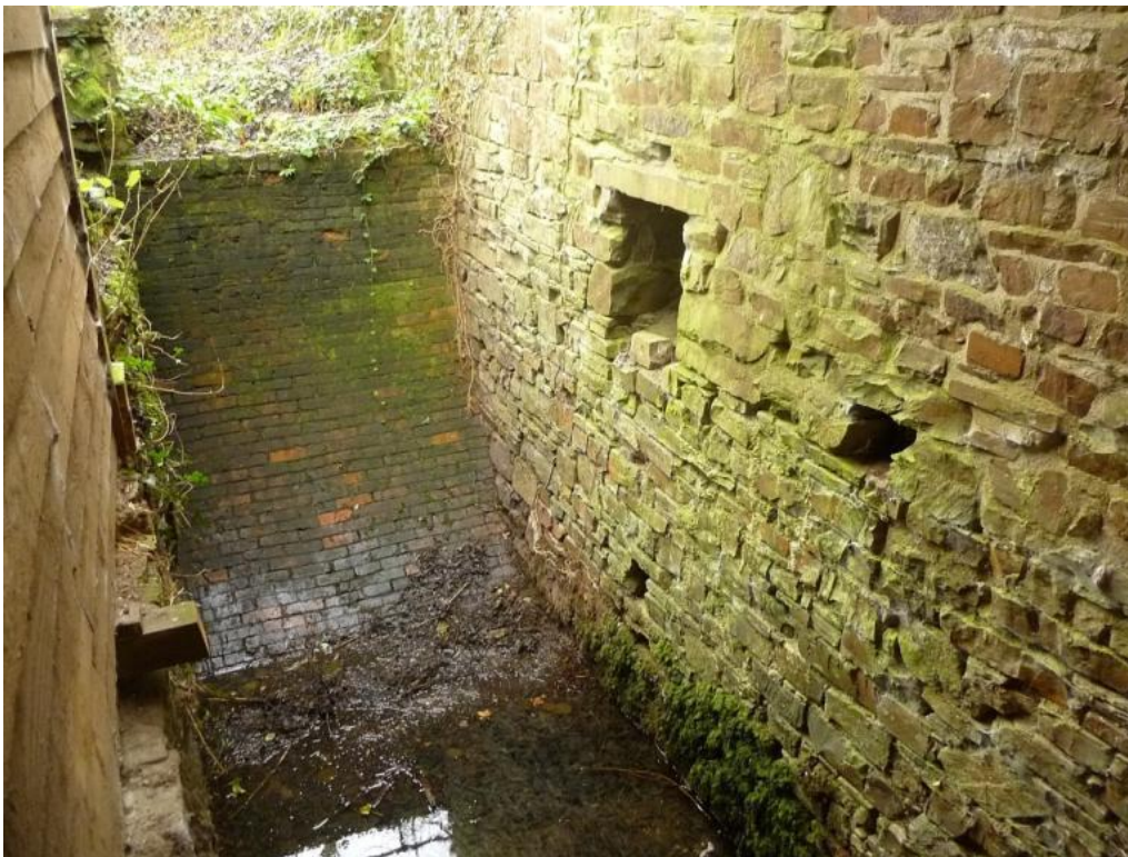
Wheelpit, showing curved brick breastwork at south end and wheelshaft opening
