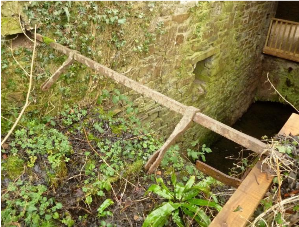
Looking down into wheelpit, with remains of penstock control
