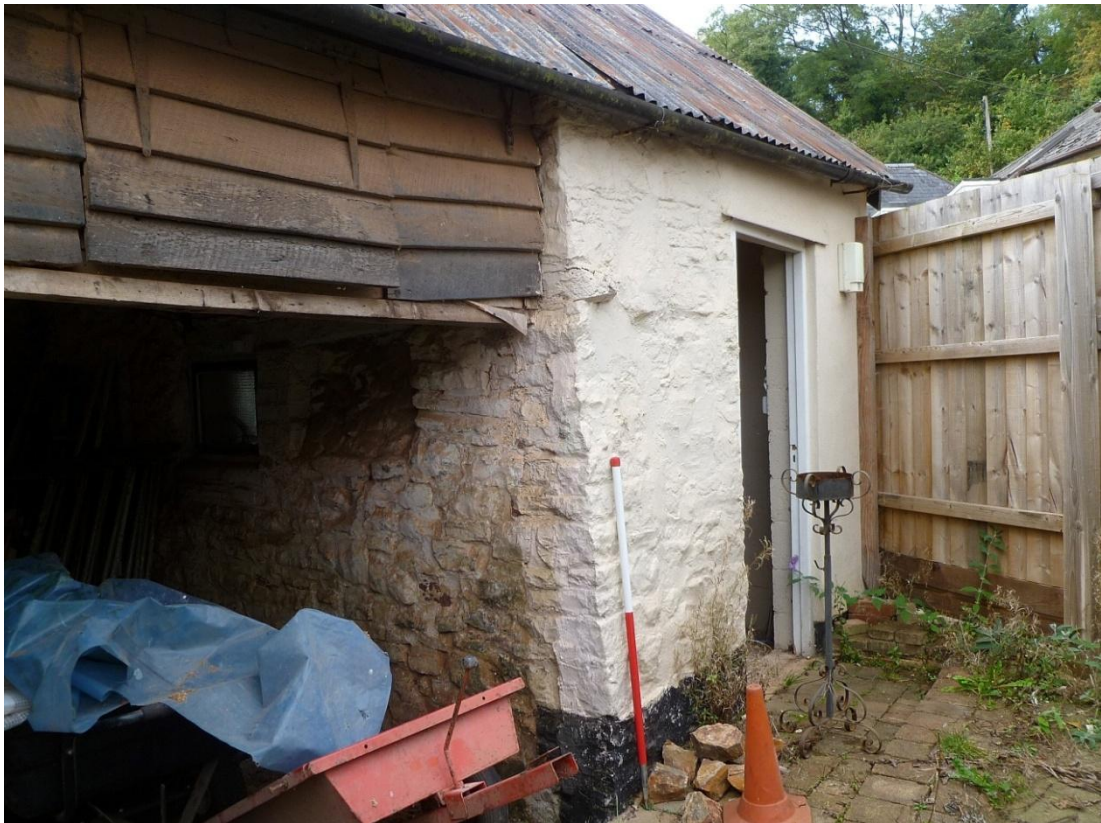
The enclosed and partly rebuilt NW end. 1m scale
