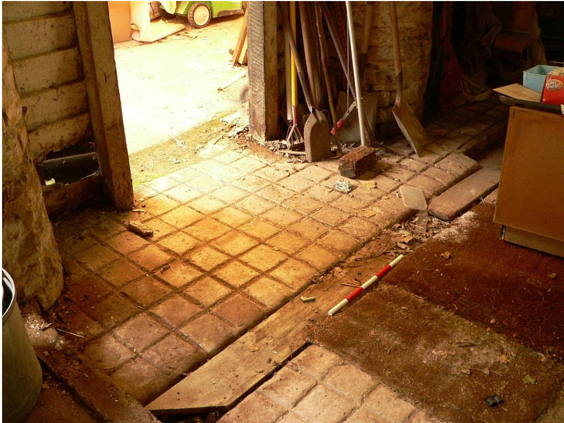
Concrete floor with tile effect and drain in bay 5. 0.5m scale
