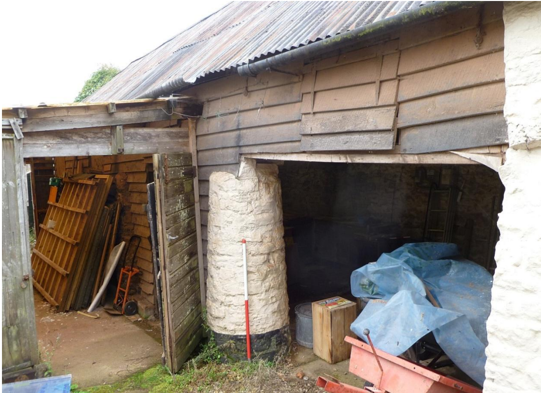
The open front of bay 5, showing one of the stone columns. 1m scale
