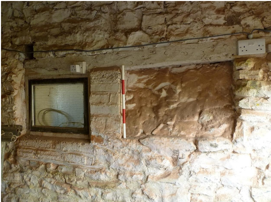
Former openings in stone wall between bays 5 and 6. 0.5m scale
