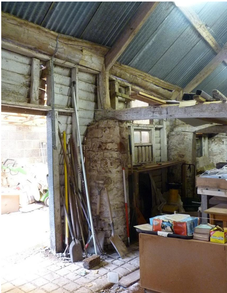
Interior of bay 5, looking E
