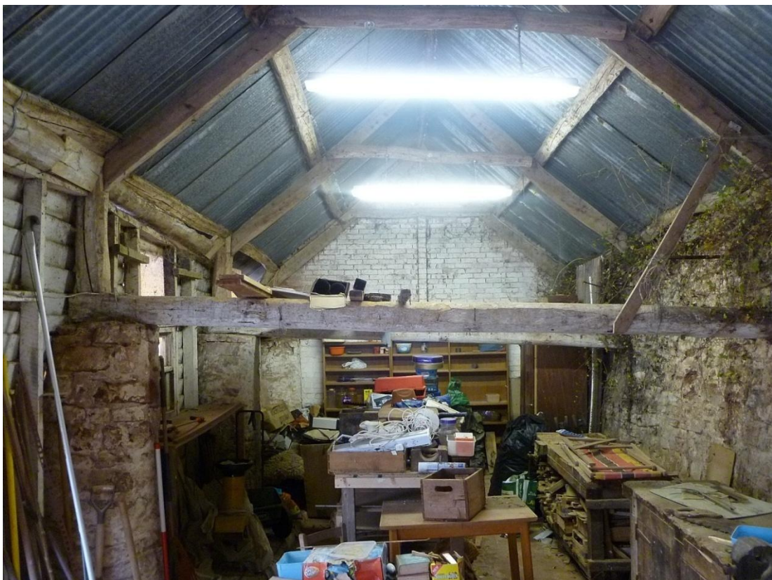
Interior, looking SE from bay 5
