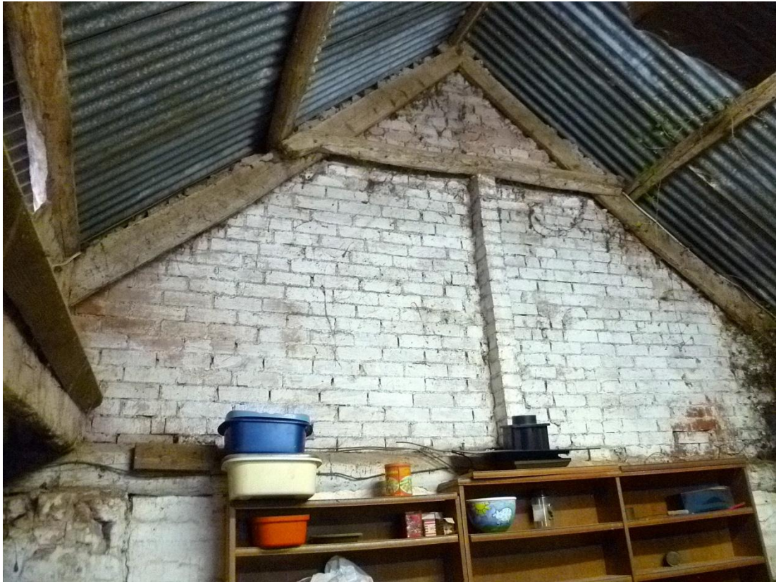
Inserted brick wall between bays 1 and 2, from NW
