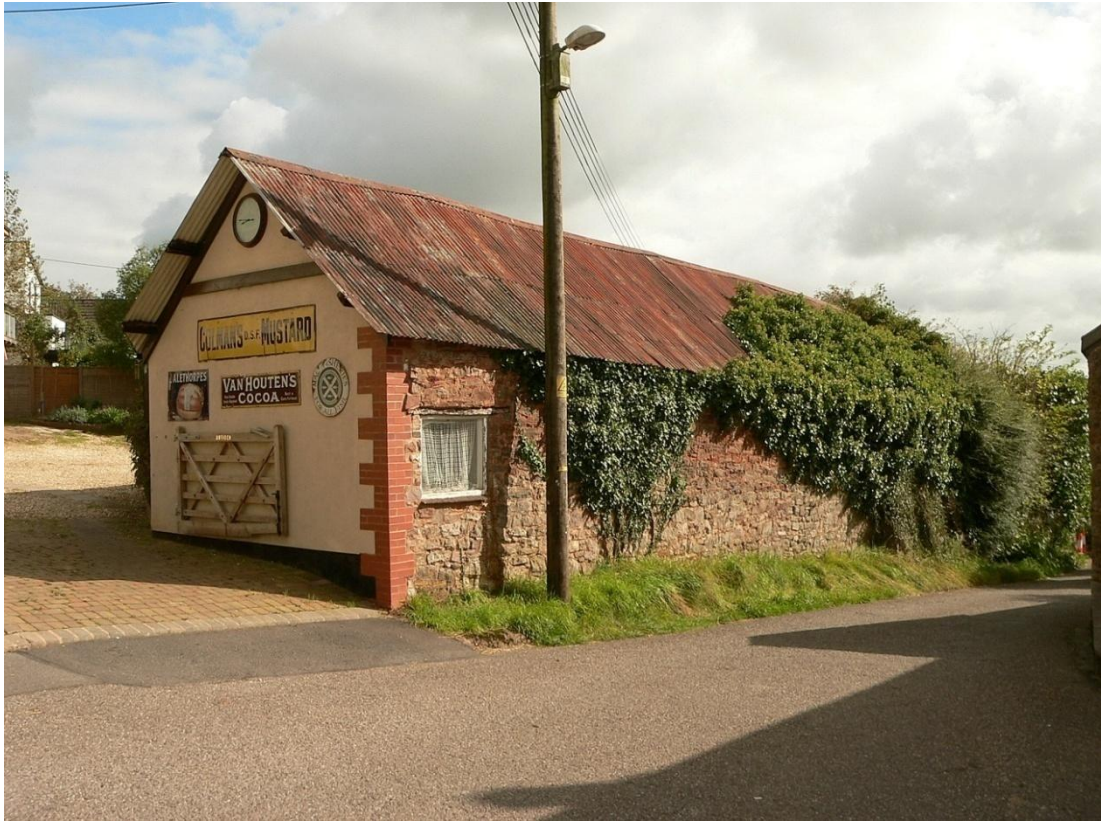
Former linhay from the north-west, showing the rebuilt NW gable end
