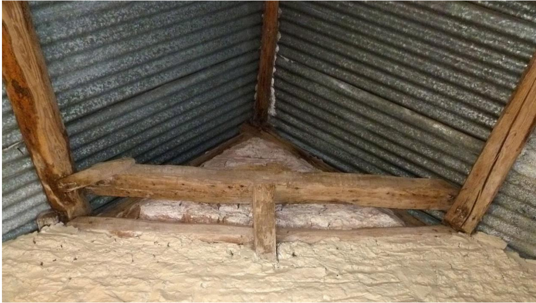
Timber between purlins at wall head between bays 5 and 6
