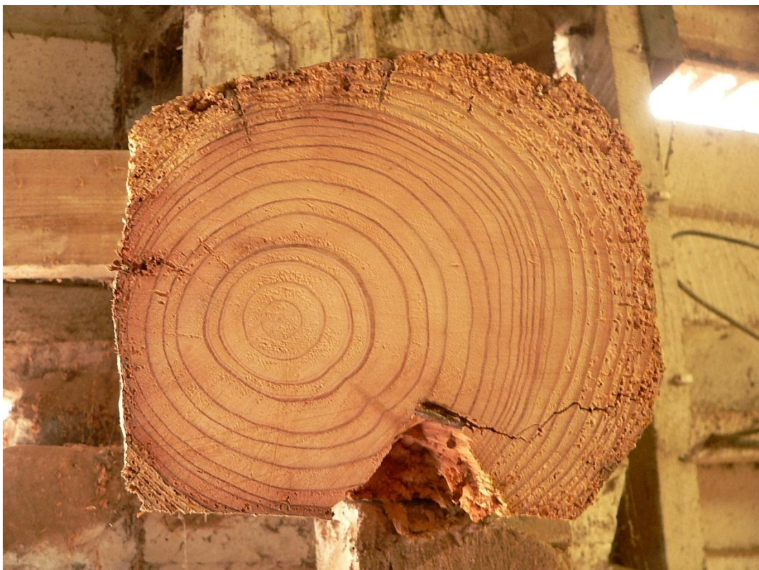
Cut end of softwood tie beam showing growth rings (25cm wide x 18cm deep)
