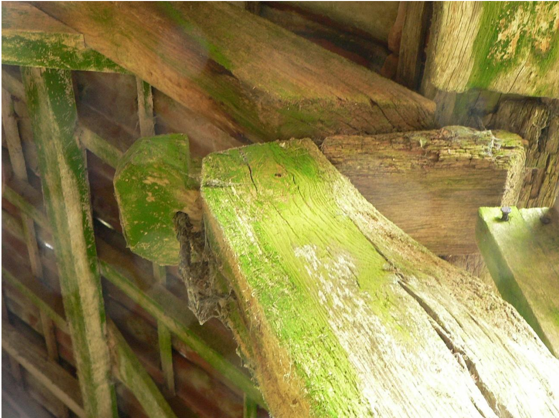
Detail of timber plate carrying foot of principal, P2, showing metal spike to left of post
