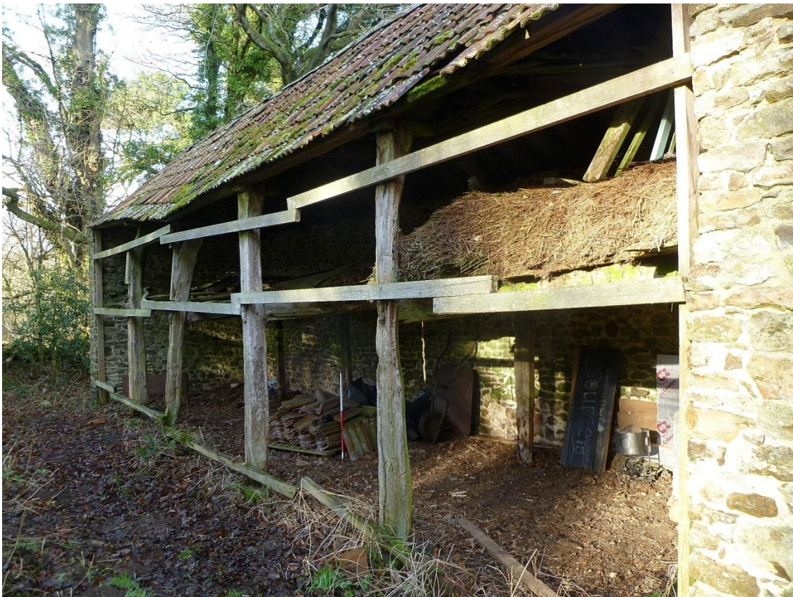
South front of linhay, looking west, showing modern bracing timbers
