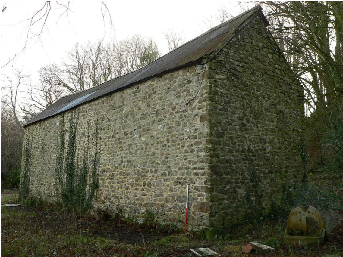
North wall and west gable, from the north west. 1m scale
