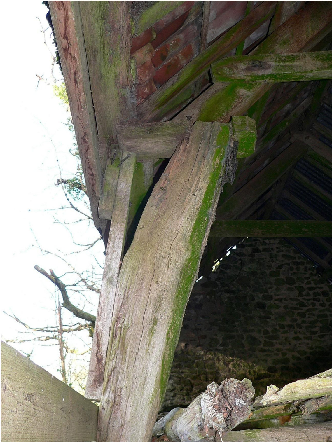
Curved head of post P1, east side, showing shaped timber plate carrying foot of principal
