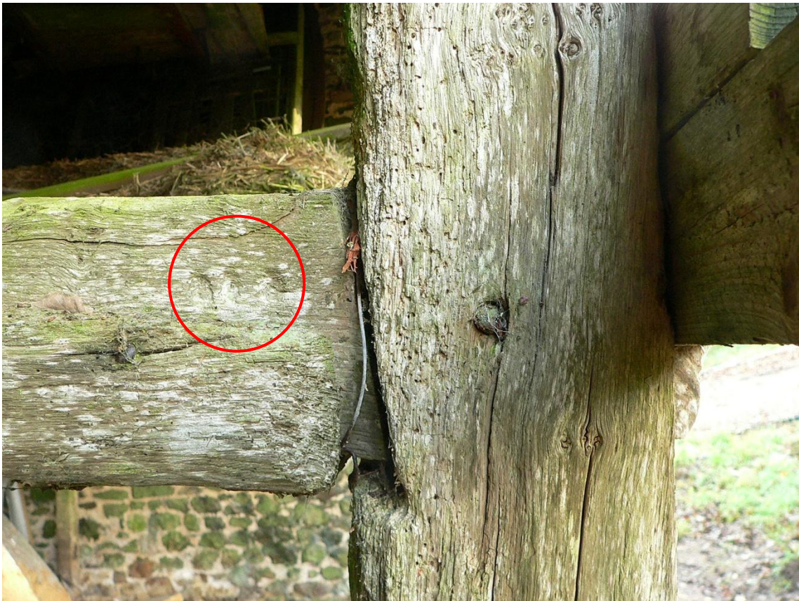
Cross beam / post joint, pegged, P3, showing assembly marks
