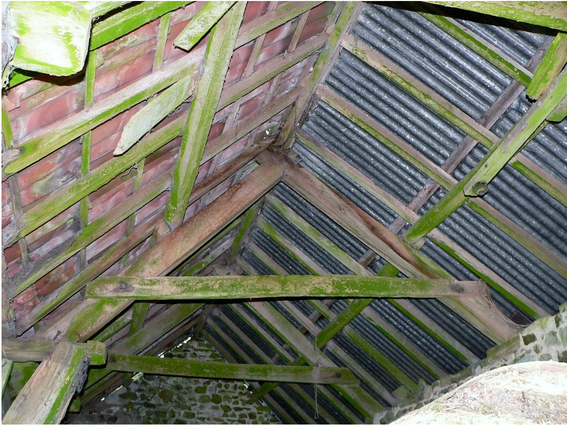
Roof structure, looking west
