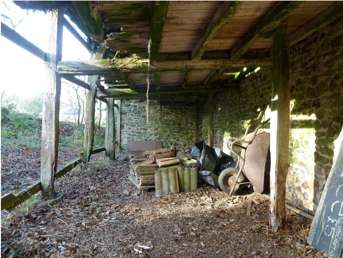
Ground floor interior, looking west, showing tallet floor structure
