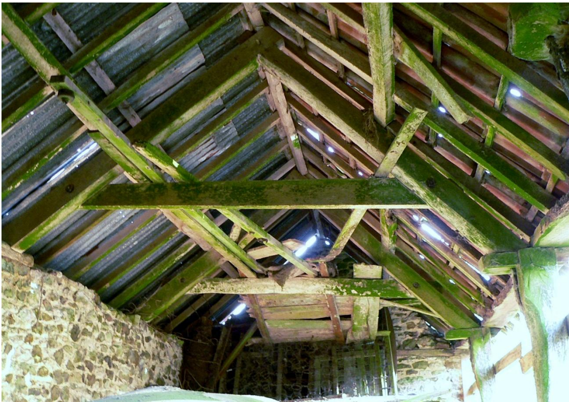
Tallet and roof looking east
