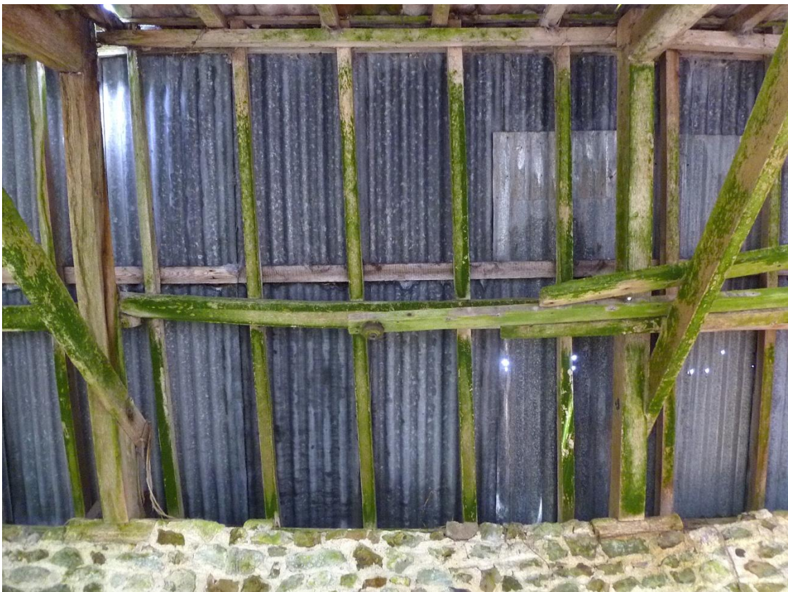
Roof construction, north slope, bay 3
