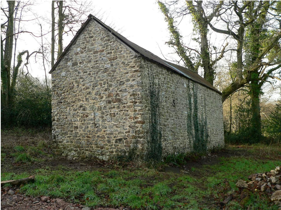
East gable and north wall, from the north east
