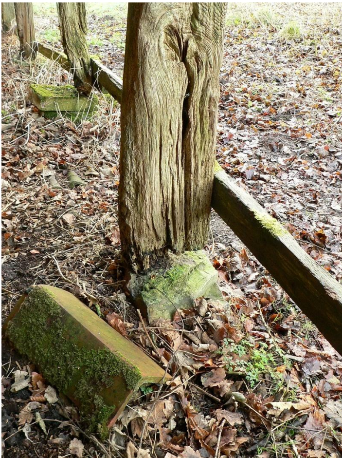
Stone bases under feet of posts
