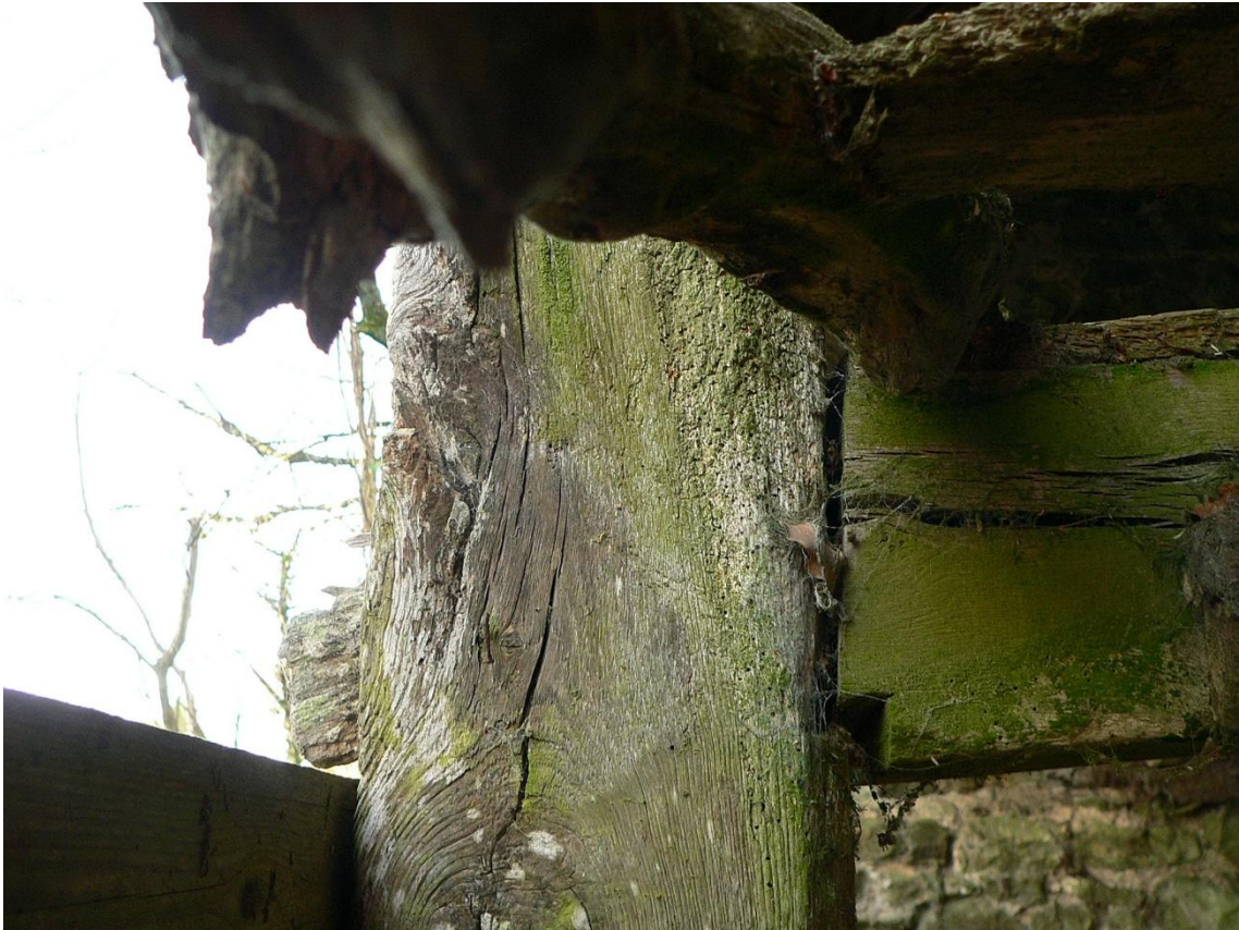
Detail of cross beam to front post joint, P1, east side
