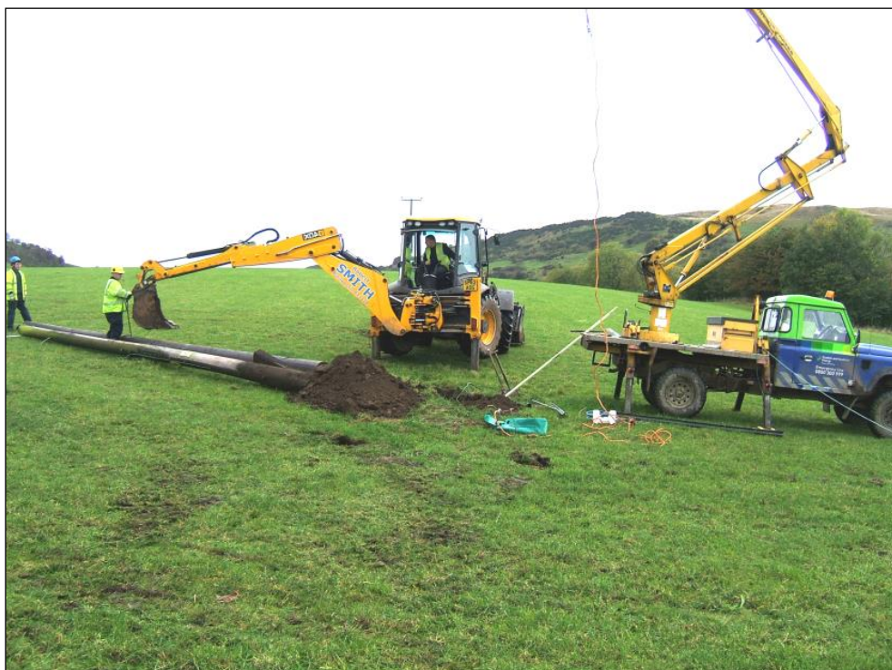
Location of the pole trench
