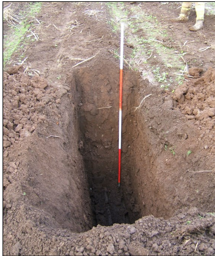
The trench for Pole 49, viewed from the east
