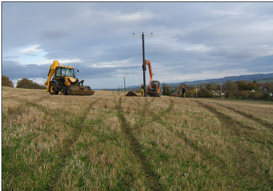
View eastwards across the west field, showing Pole 55 being erected
