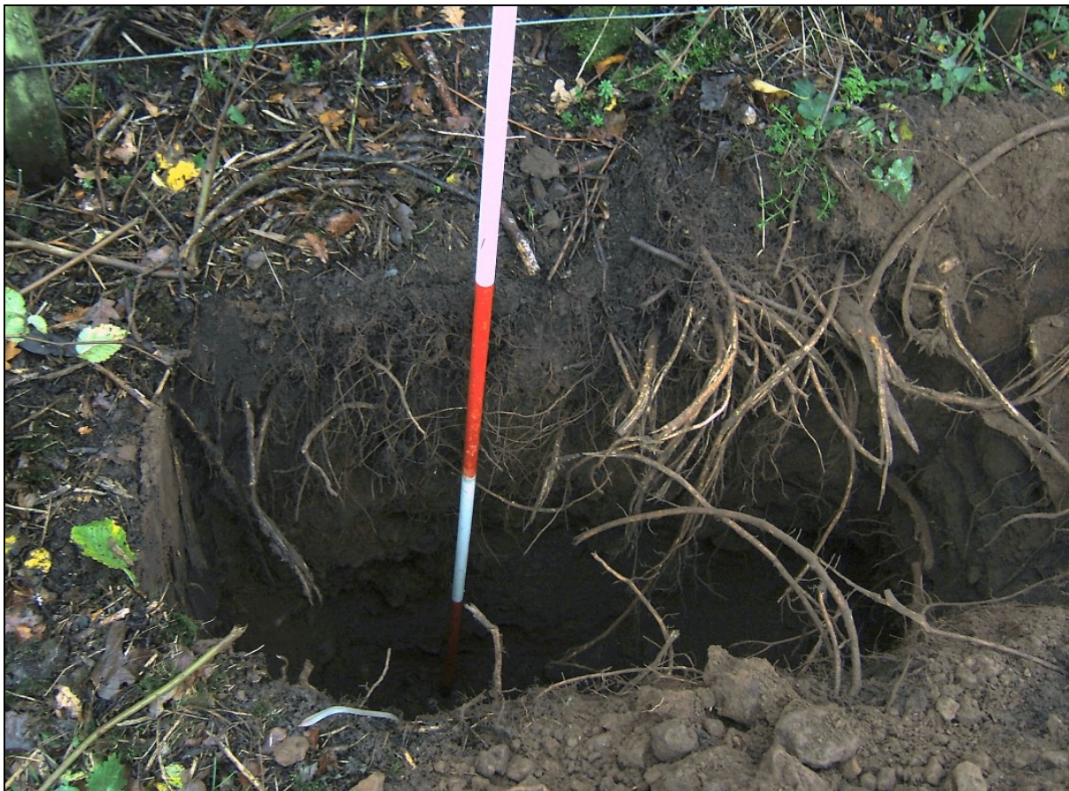
Trench for replacement Pole 2
