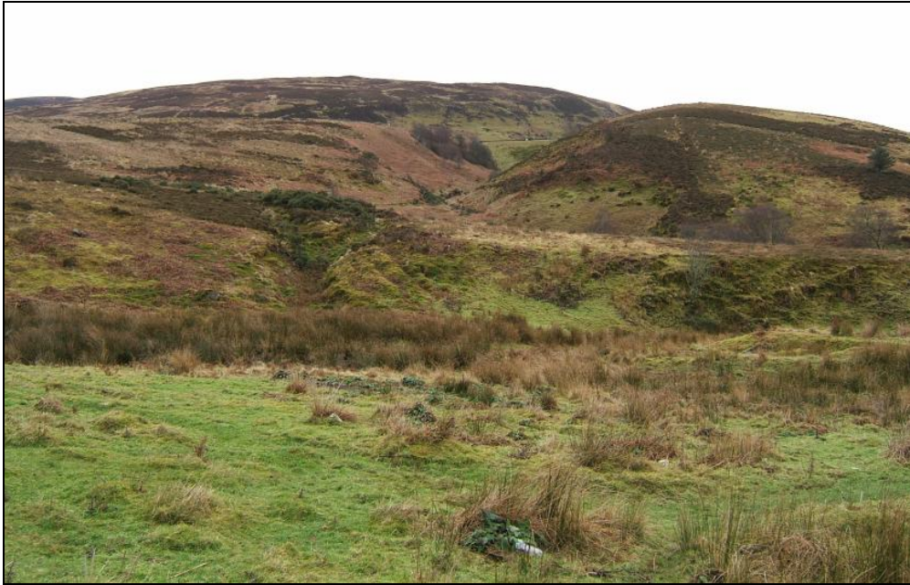
View, from the north, of the upper stretch of the penstock
