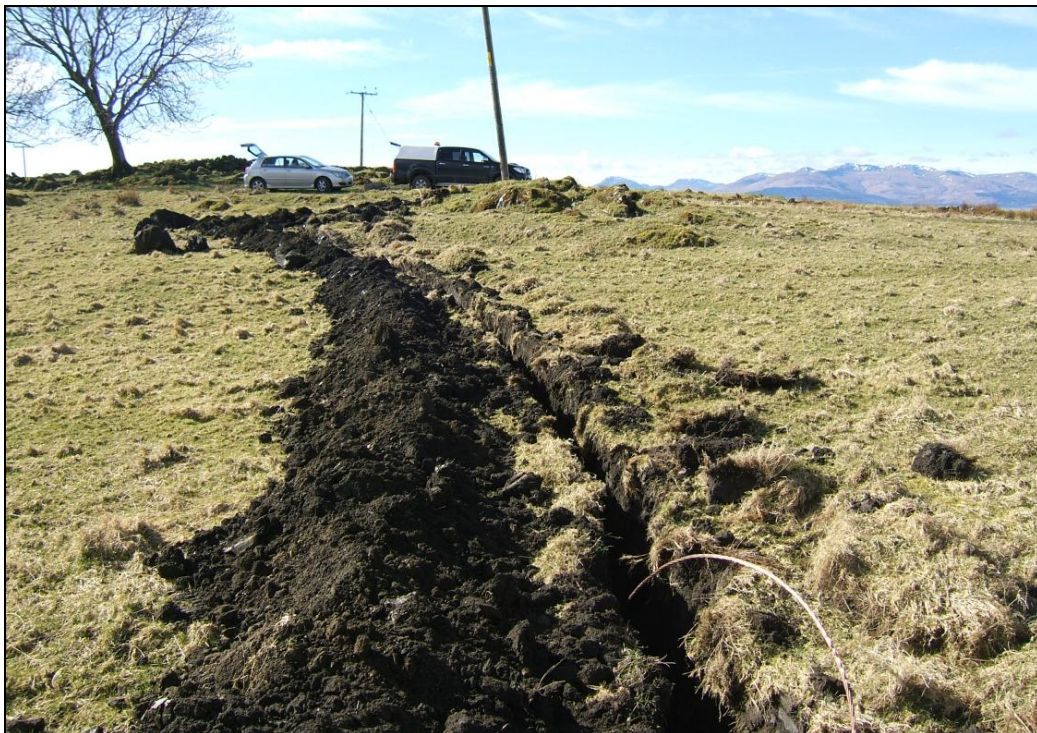
Trench viewed from the north-east
