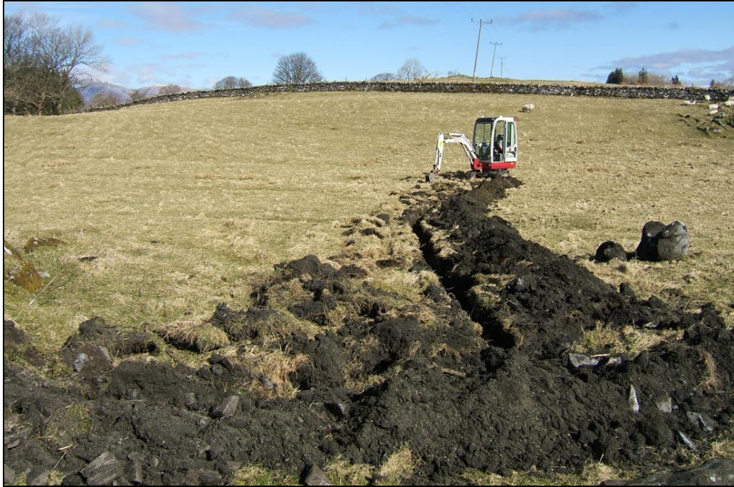
Trench viewed from the south-west
