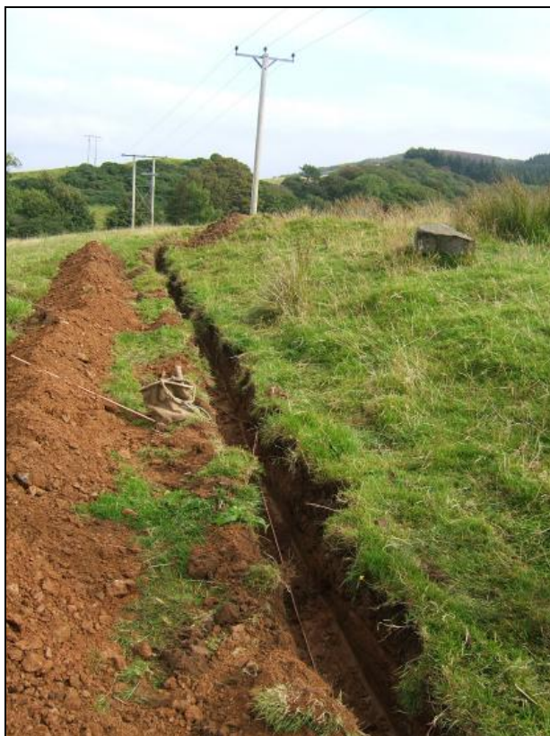
Earth wire trench and Pole 23, viewed from the south
