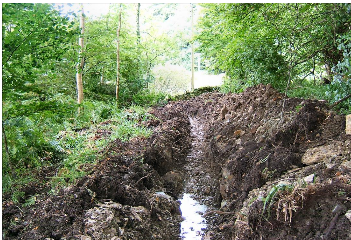
West end of trench with Pole 1 in the distance
