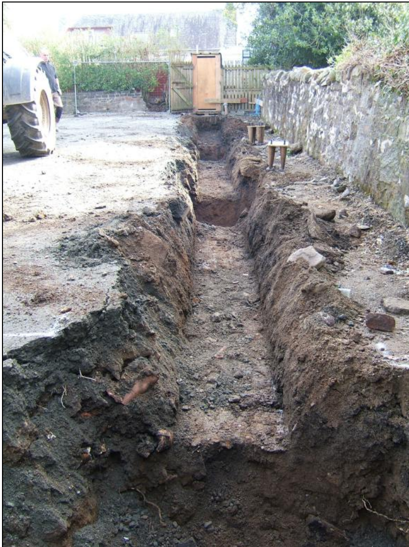
South trench viewed from the west
