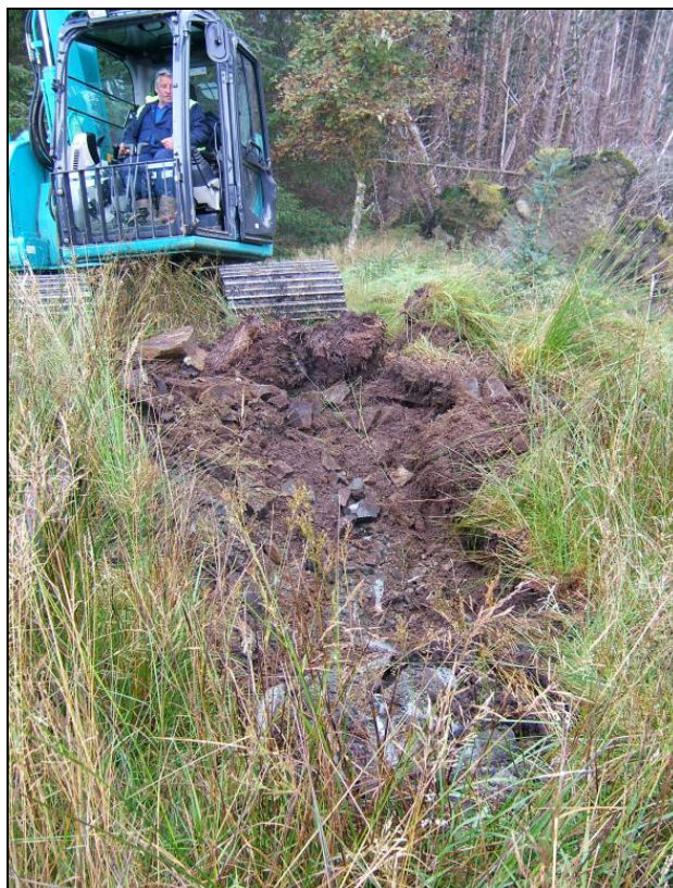
Pole 13 stay trench, showing exposed bedrock
