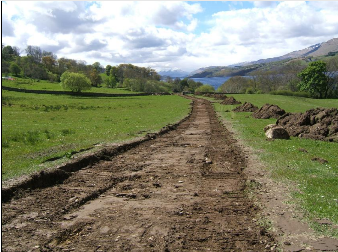
Access road trench, viewed from the east
