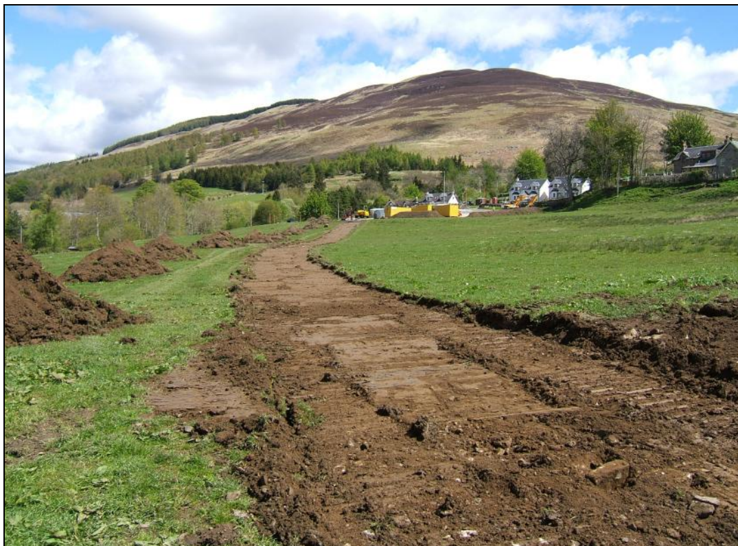
Main trench looking towards the contractor's trench from the west
