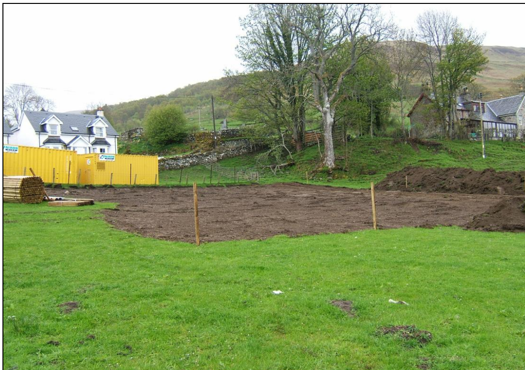
Site of the contractor's compound, viewed from the north
