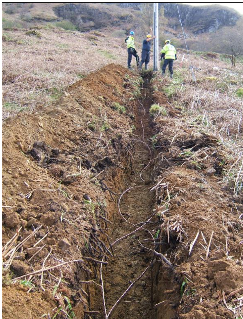
Earth cable trench, viewed from the west
