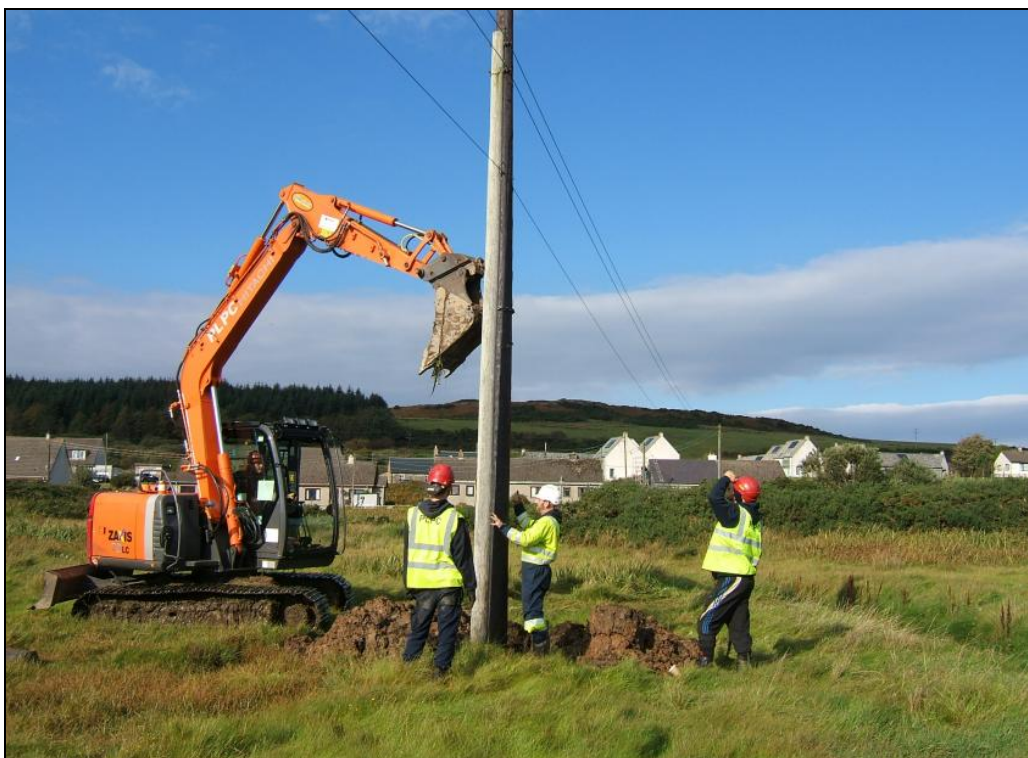
Replacing Pole 5 in Area M
