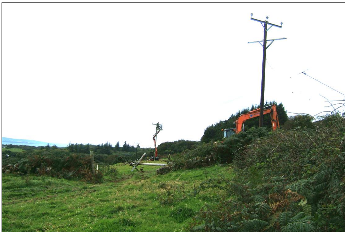
Area K: new Poles 17, 18 and 19 being inserted; viewed from the north
