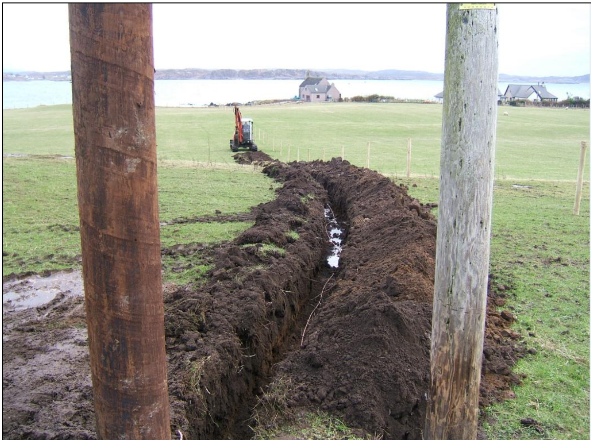
Earth-cable trench running downhill from Pole 25; viewed from the north-west
