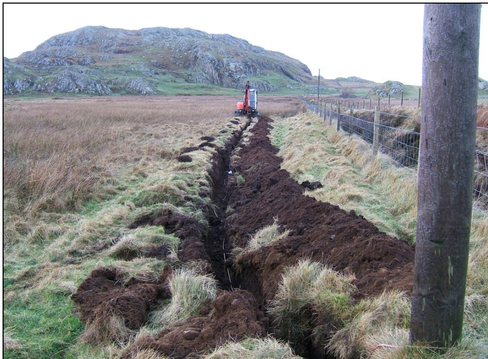
TAG trench for Pole 15, viewed from the south
