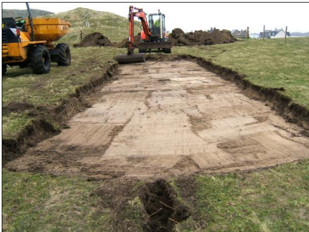
Trench for the septic tank and soakaway, viewed from the south-west
