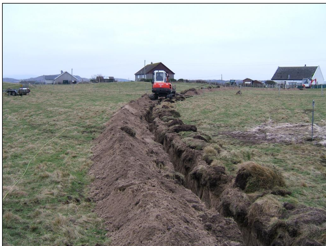
Cable trench being excavated; viewed from the west
