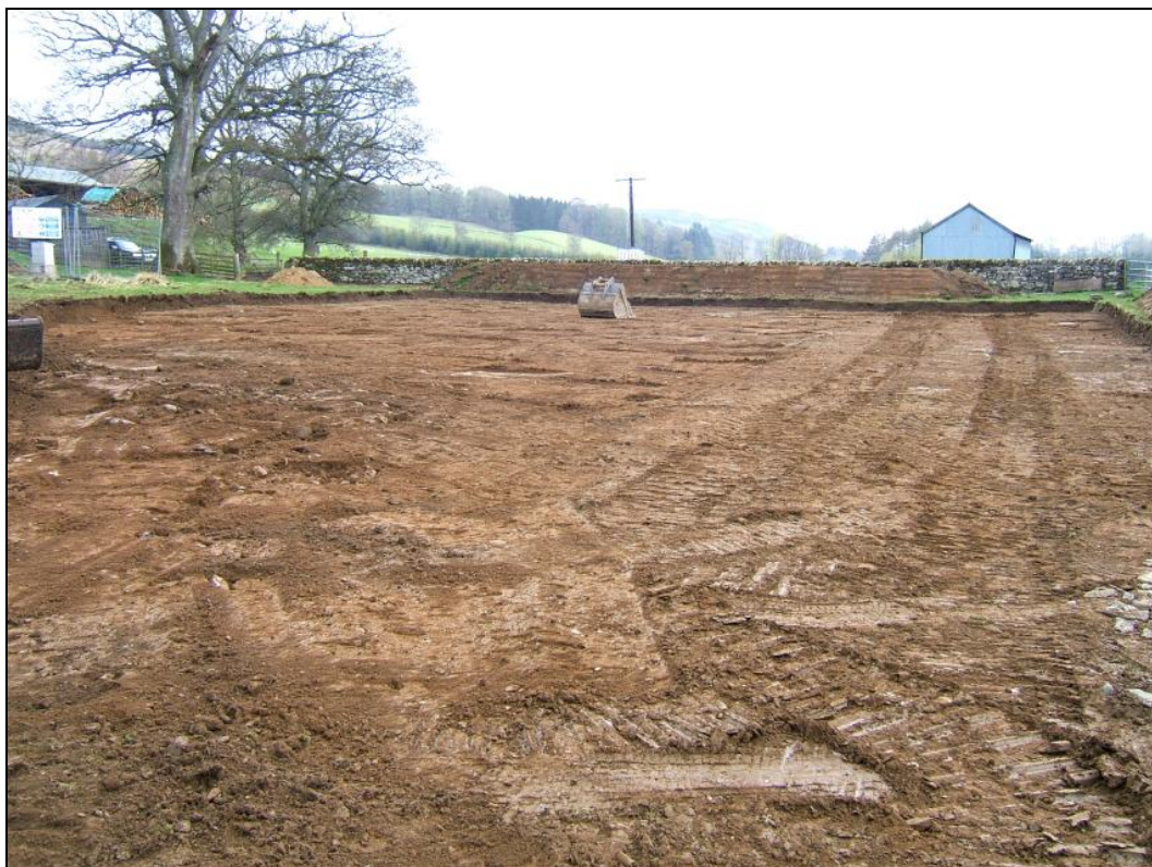
The site stripped of topsoil, viewed from the north-east
