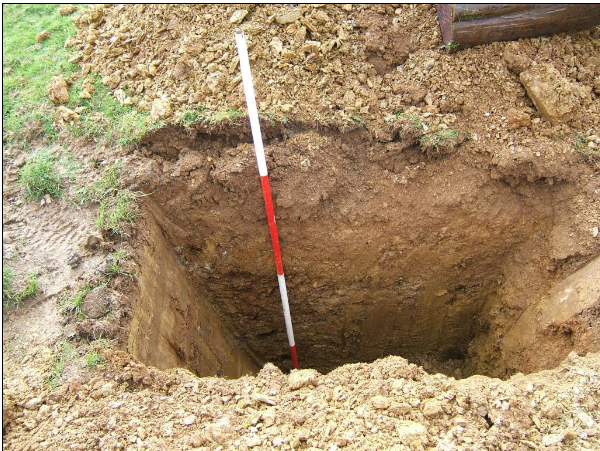
Trench for the new Pole 72, viewed from the north-west
