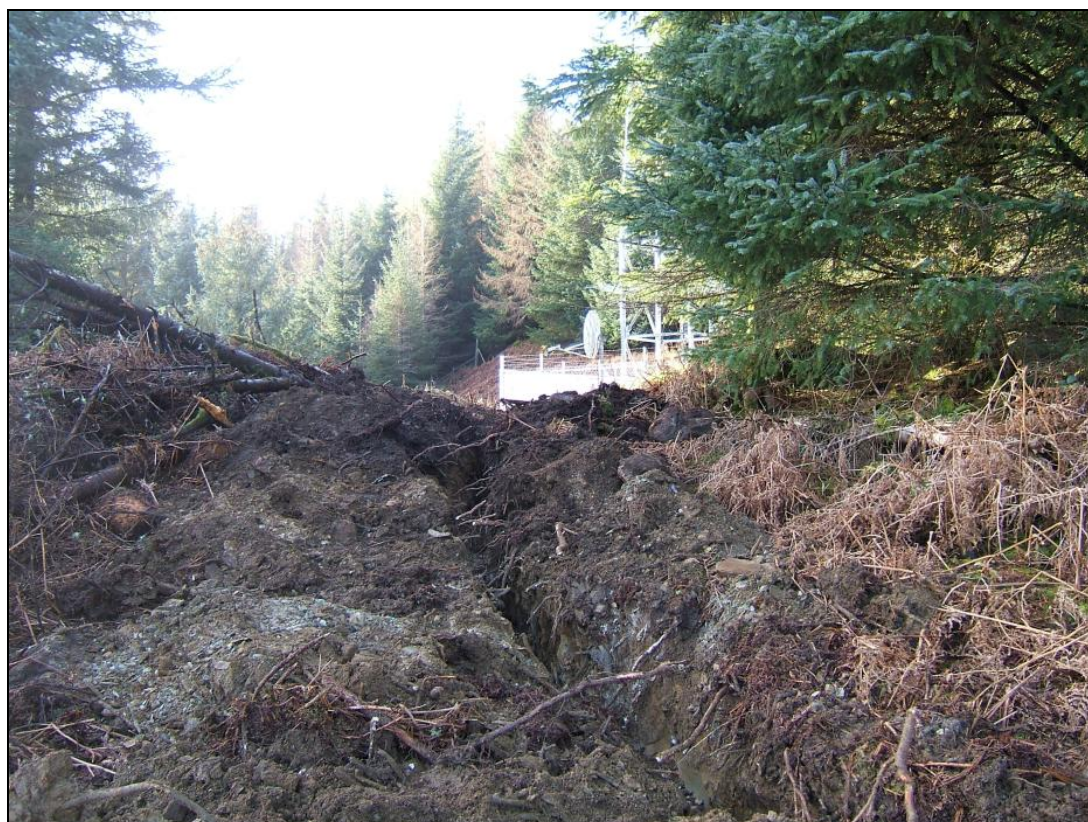
The cable trench approaching the EE mast, viewed from the east
