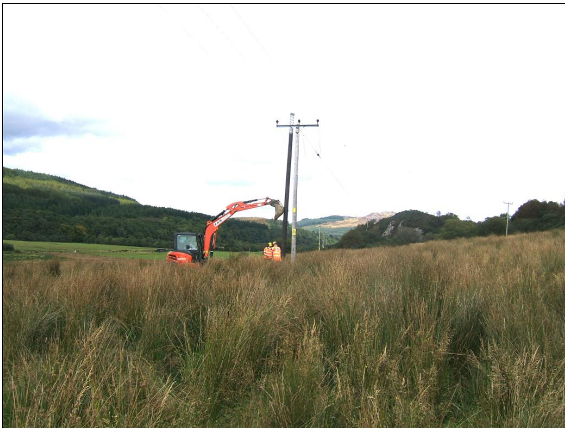
View northwards up the Kilmichael glen showing Pole 2 being erected
