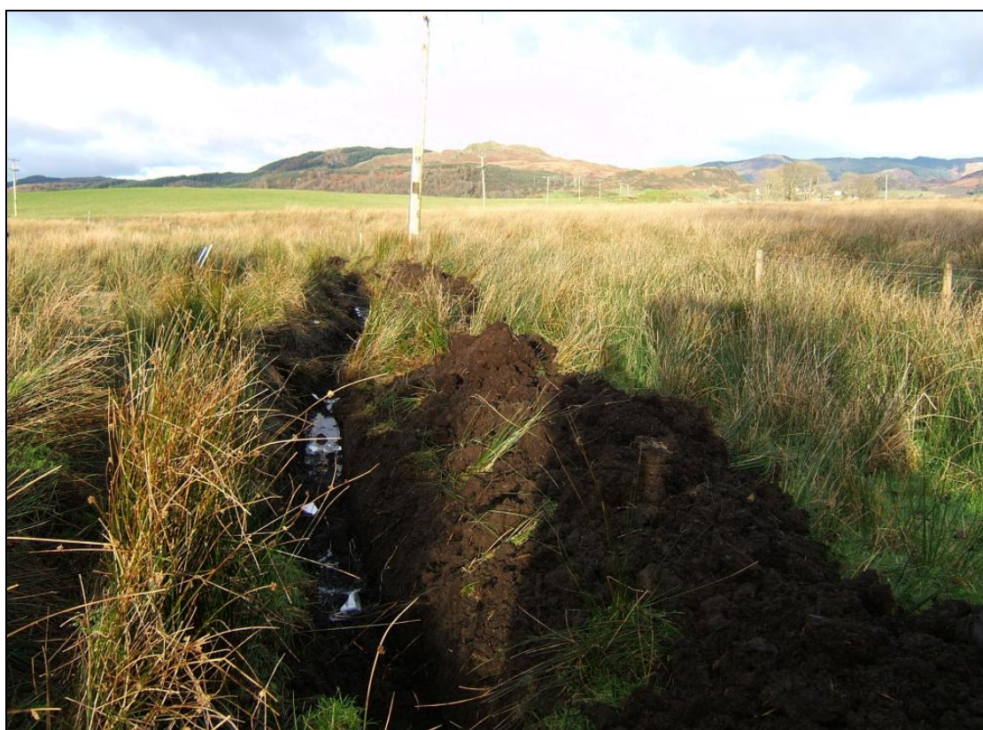
Pole 49 and the earth wire trench viewed from the south
