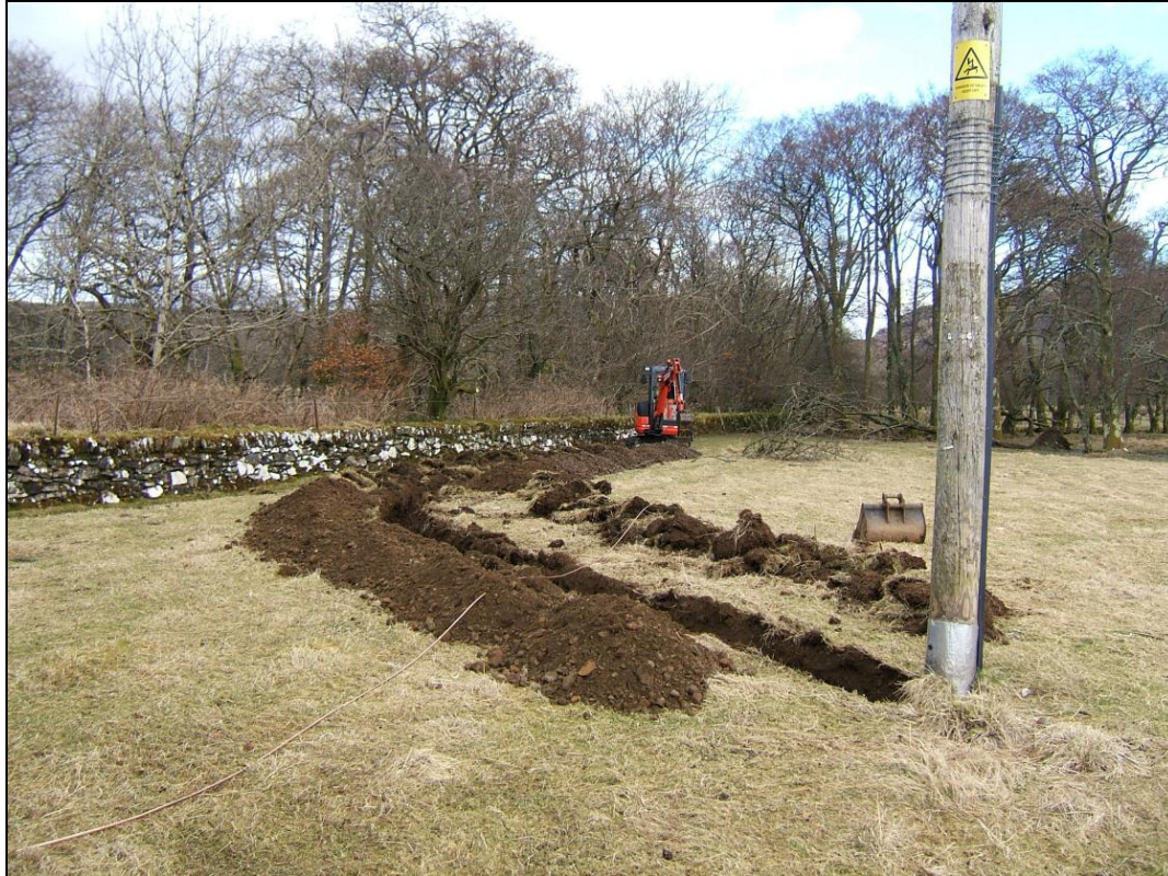
Trench at Pole 152 viewed from the west
