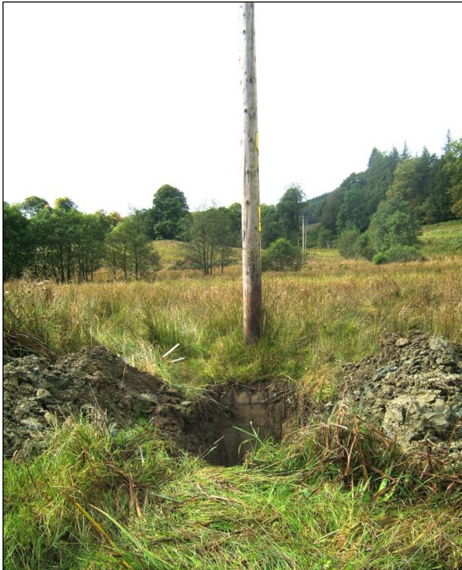
Old Pole 19 and trench for its replacement, viewed from the east
