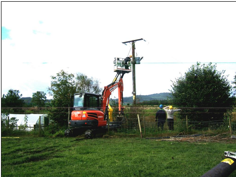
Old Pole 48 being dismantled
