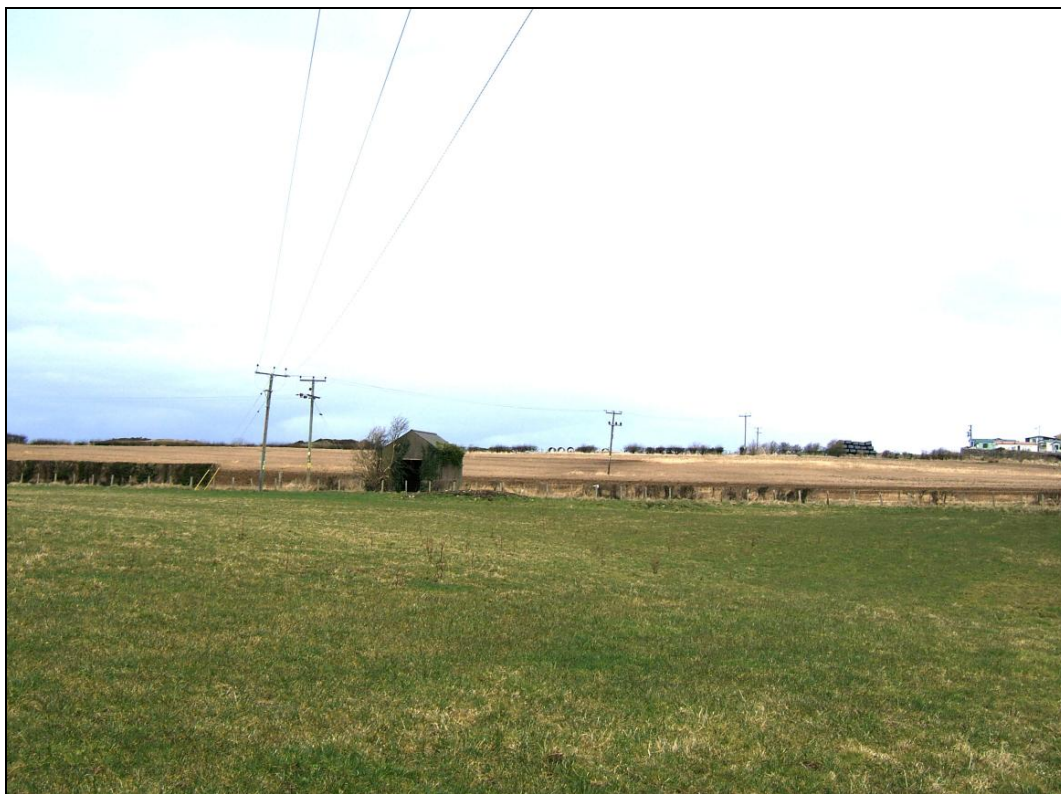
View to the north-west from near the south-east terminus of the overhead line
