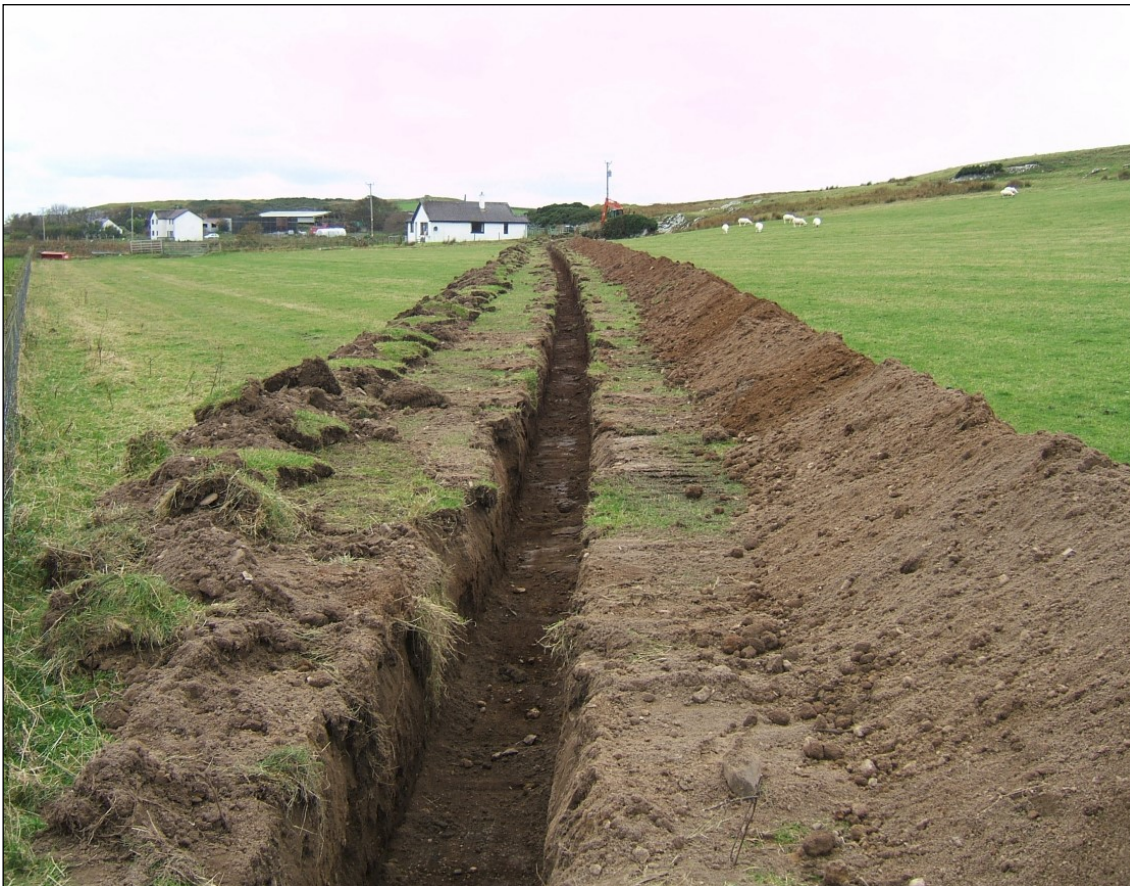
View of the trench from the south-east looking towards Pole 17
