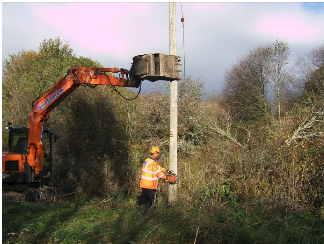
Pole 14 being cut 1m above ground
