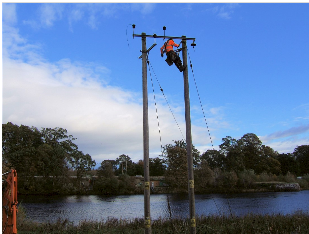
Dismantling metalwork on Pole 17
