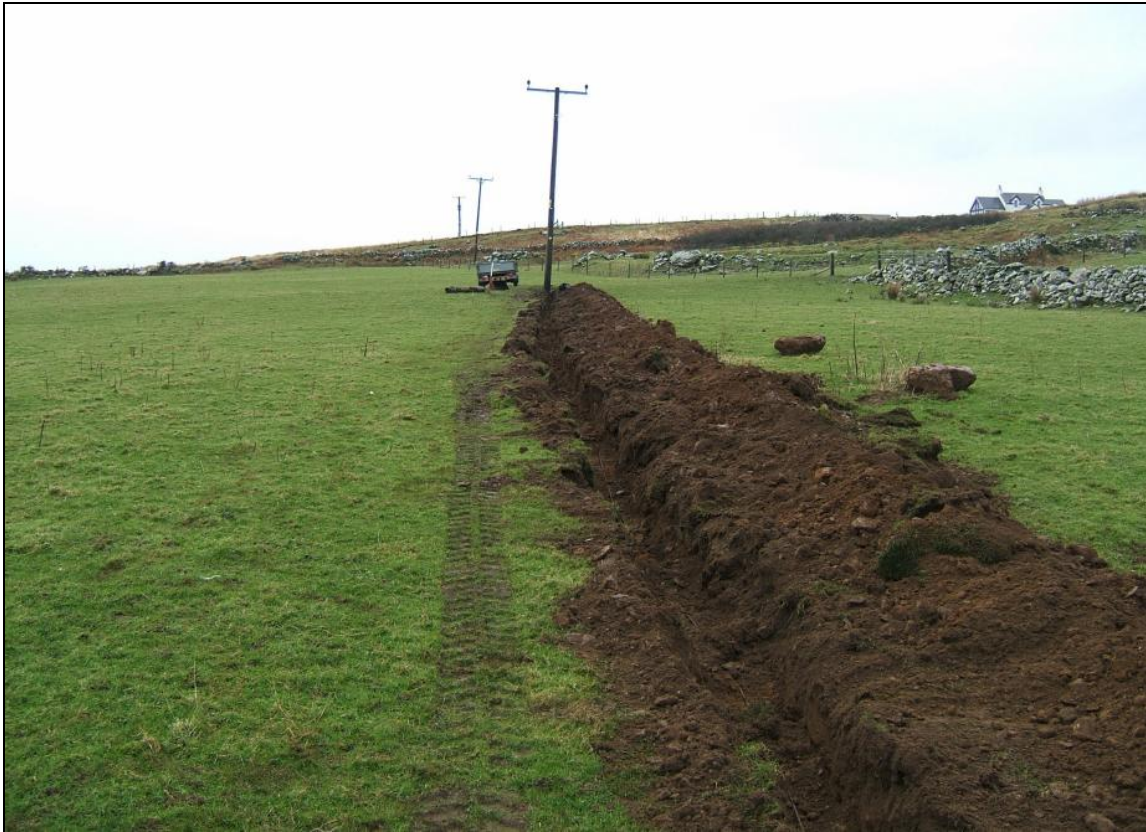
Earth wire trench looking northwards to Pole 31
