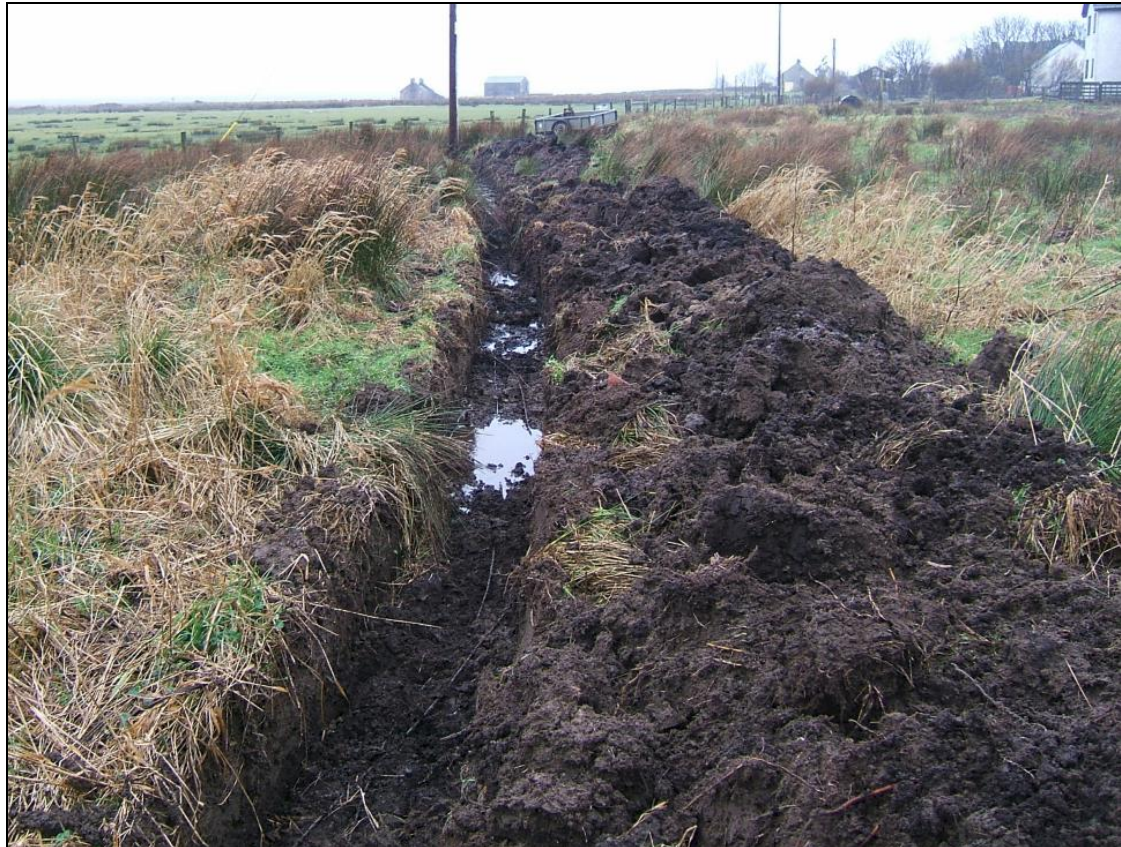
Earth wire trench looking westwards towards Pole 18
