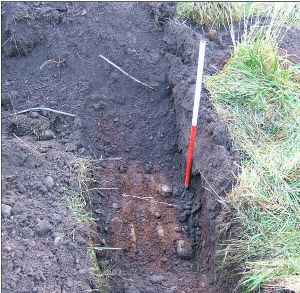
Trench for Pole 28, viewed from the north-east
