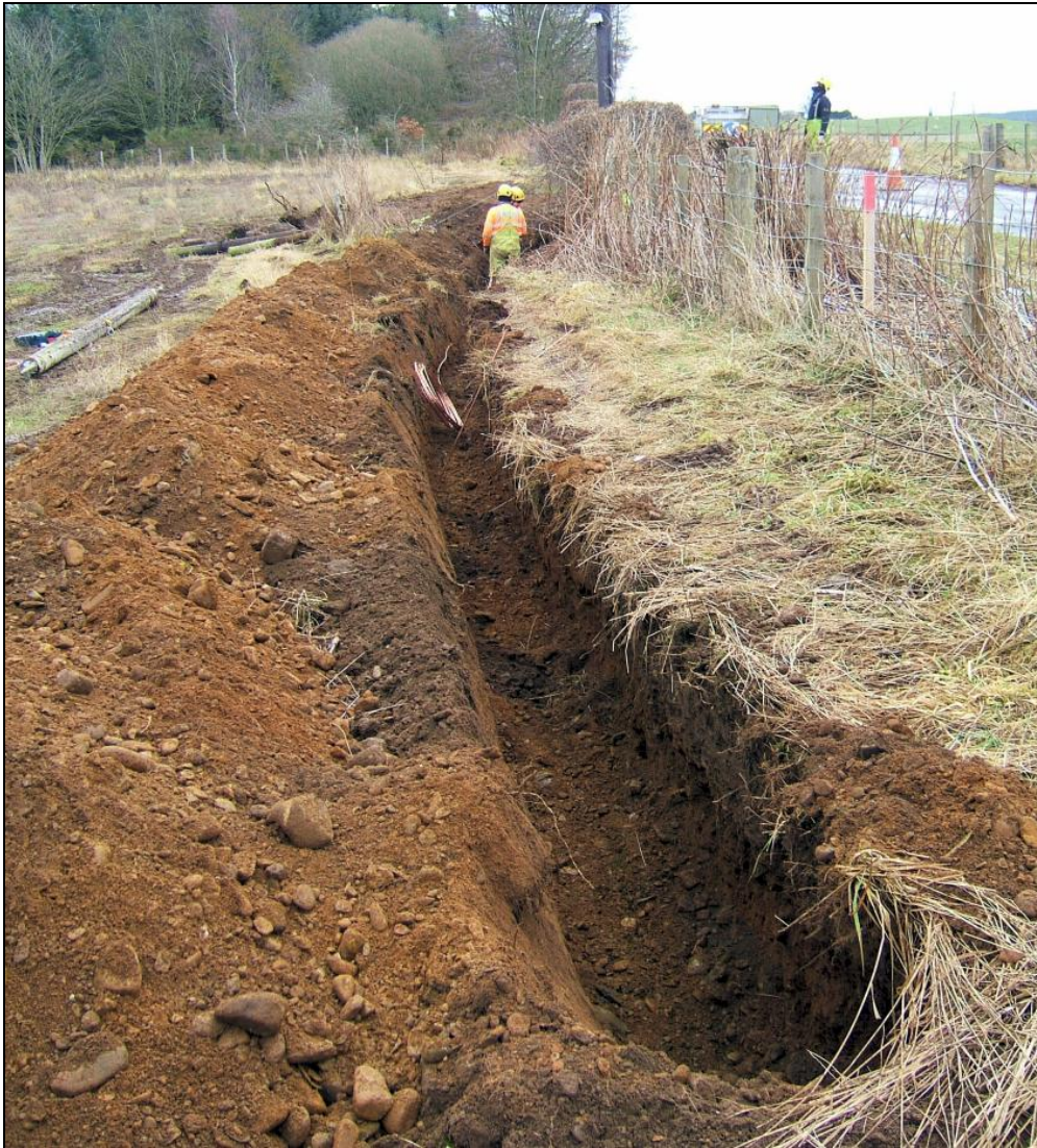
View, from the west, of Earth Wire Trench 2
