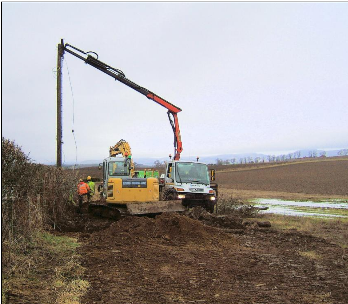
View from the east of Pole 7 being replaced
