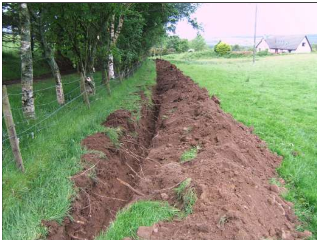
Cable trench from the south-east
