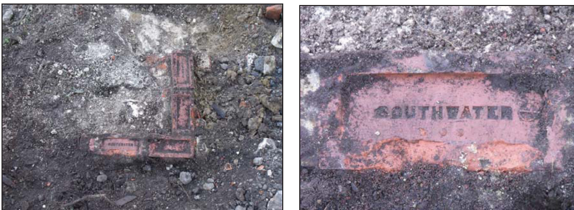
Fig 3 The foundations of the demolished building in the former stable yard, looking northwest, and detail of the bricks used in its construction
