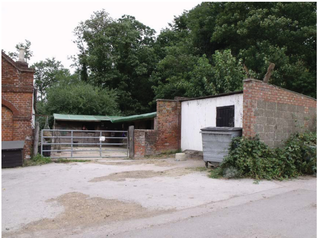
Figs 8c & d Barwell Court Farm, Chessington: views of southwest end of brick stable block and yard with buildings
